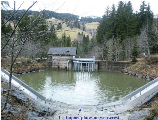
Figure 12. Impact plate array for measuring bedload transport in the Erlenbach stream, Switzerland (downstream view, with plates visible in the foreground). Geophone sensors are mounted underneath the steel plates at the crest of the large check dam. Photograph courtesy of Dieter Rickenmann.
