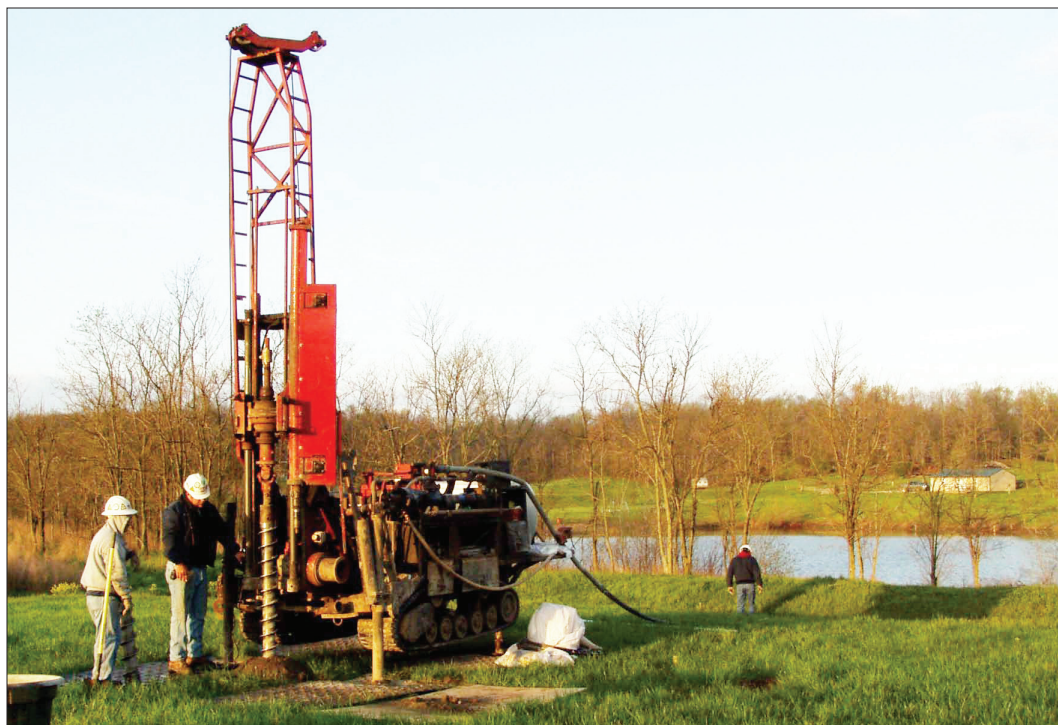
Figure 4. Drilling activities for installation of a temporary network of monitoring wells at the study site in east-central Pike County, Ind.
