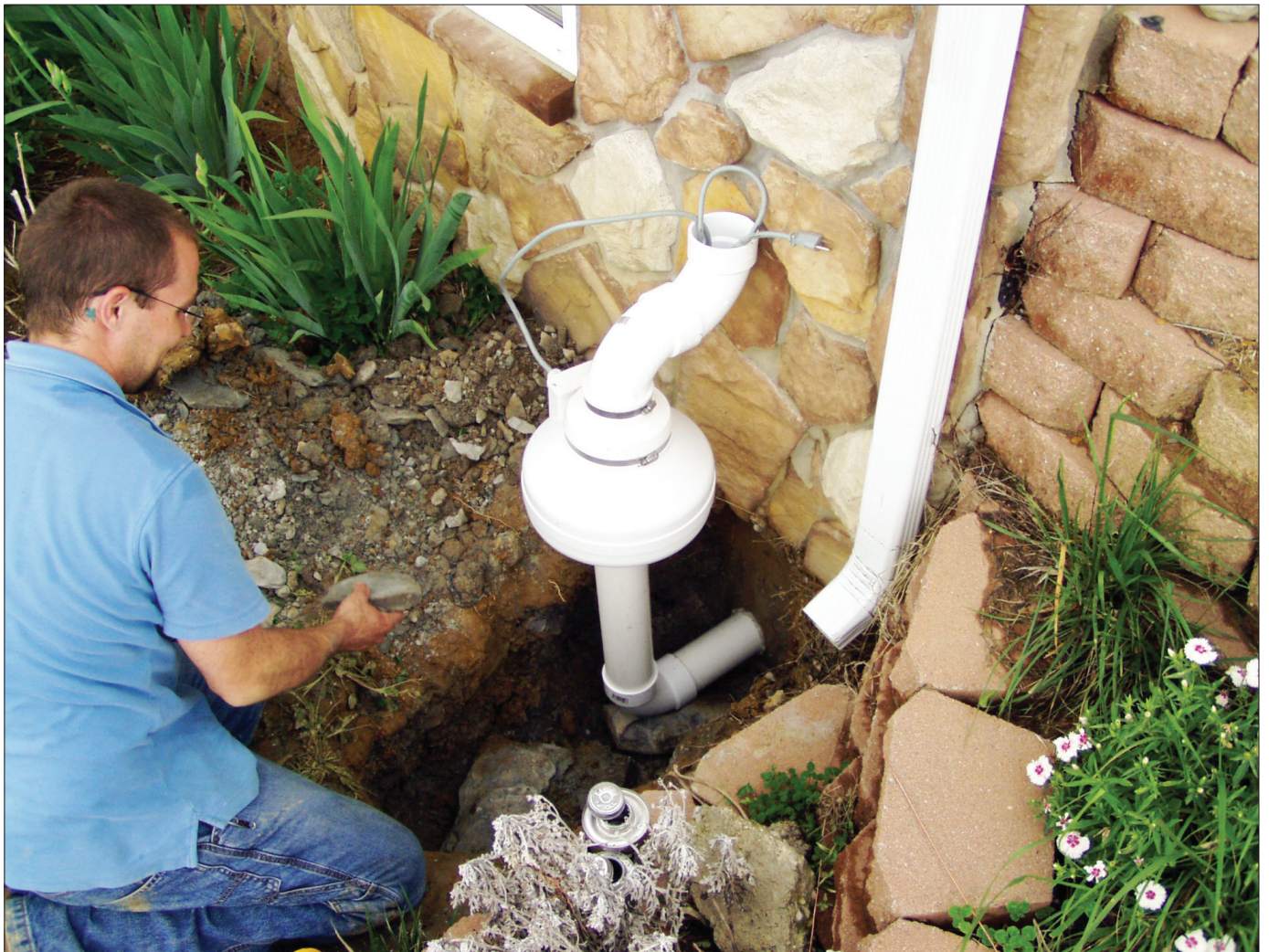
Figure 10. Mitigation system established to depressurize the block walls of the study-site home, Pike County, Ind.
