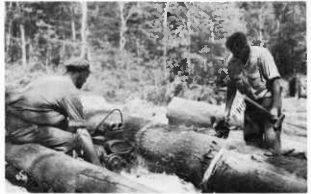
Figure 166.— Bucking at the landing promotes integrated logging.
