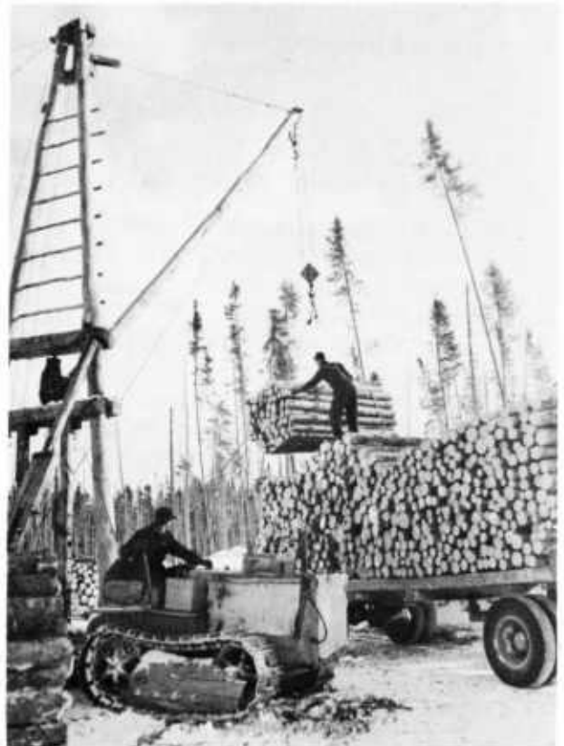
Figure 269. — Loading with a cable sling. (Courtesy Caterpillar Tractor Co.)
