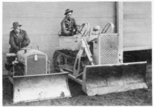
Figure 216.—Two new light tractors developed by the Forest Service. Left, the "Trail Beetle"; right, the airborne trail tractor.
