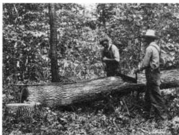
Figure 158.—Cutting a log at a crook.
