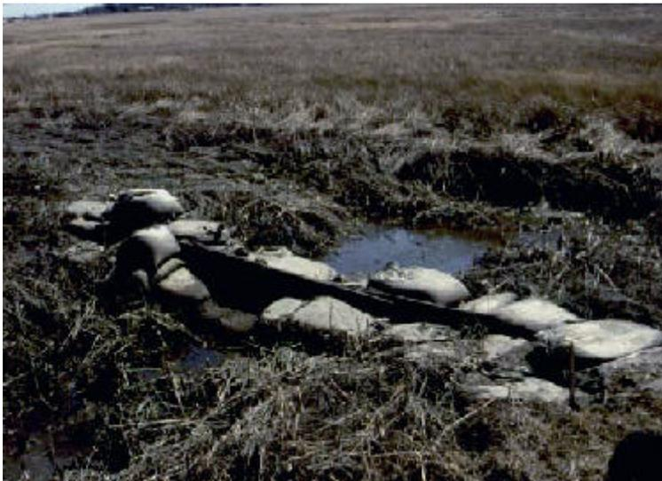
**Figure 11. Ditch plug in an OMWWM system.**
