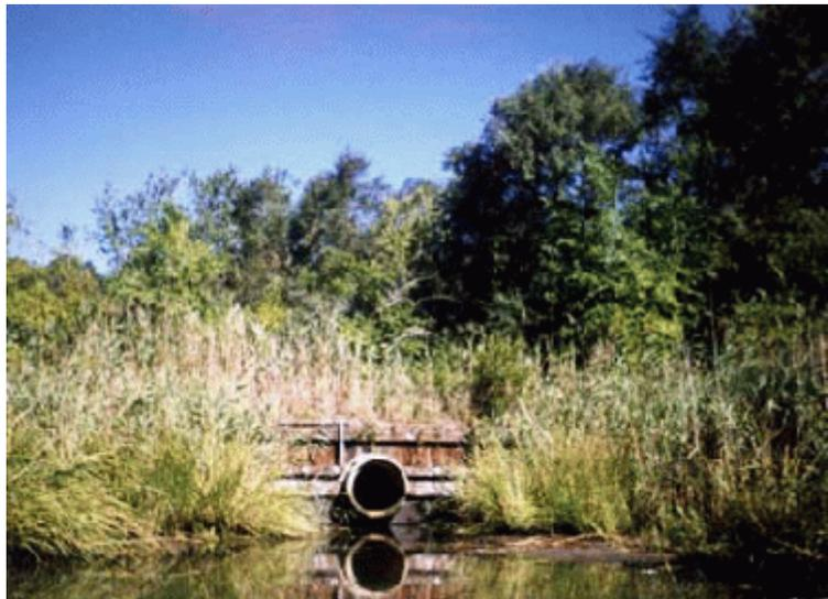
**Figure 7. Perched culvert impeding tidal flow.**
