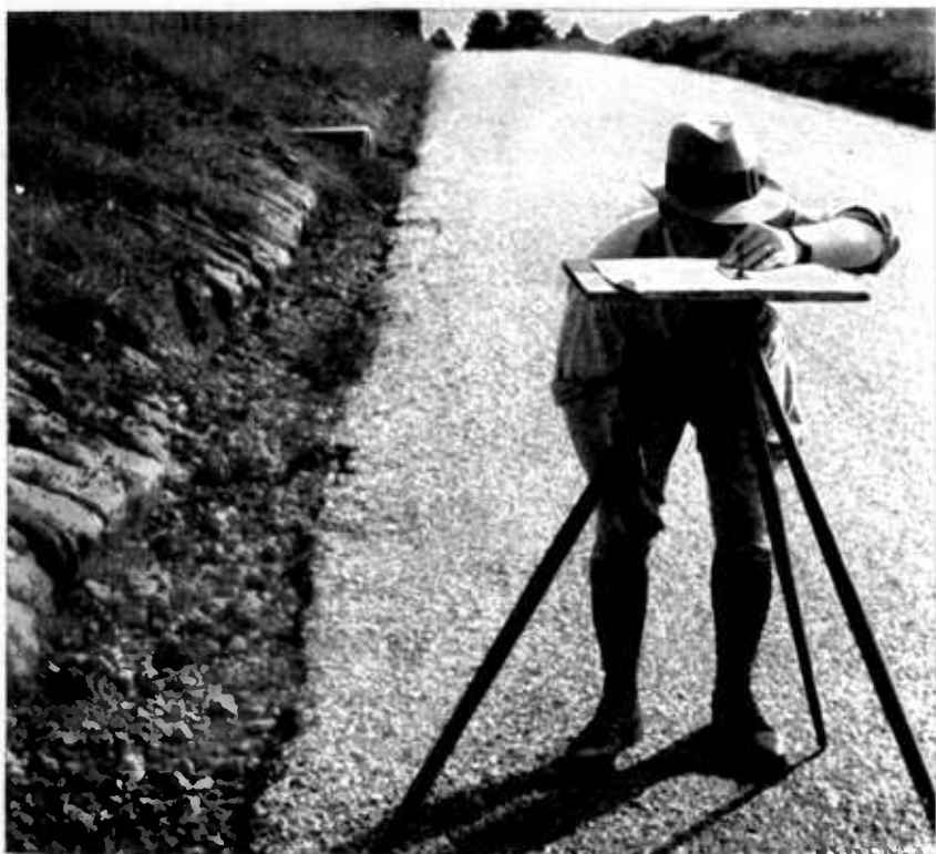
FIGURE 57.—Plane table assembled for use.
