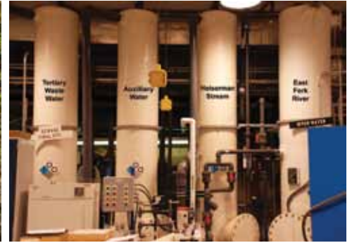
ESF water supply tanks
