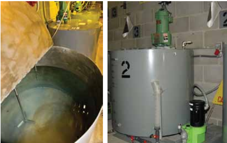
Chemical dosing tanks
