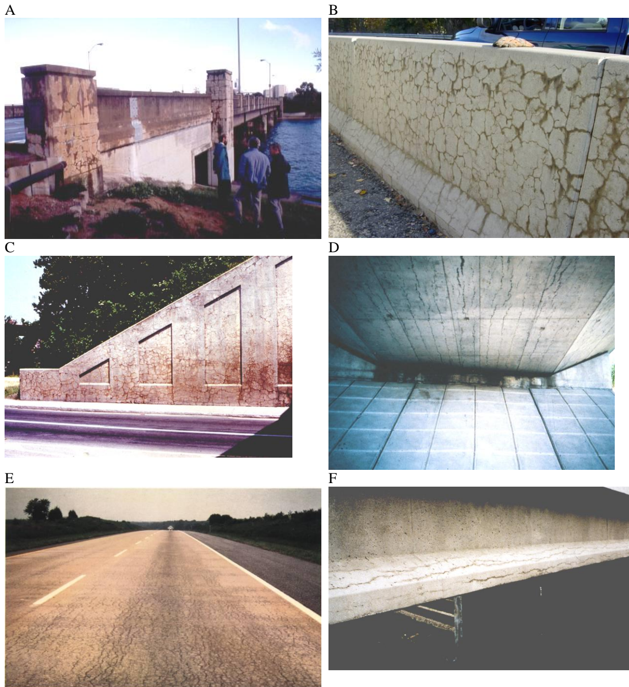
Figure A3. (A). Map-cracking in parapet walls of a bridge structure affected by ASR. (B). Severe map-cracking and associated gel staining around cracks in a median highway barrier affected by ASR. (C). Severe map-cracking in the wing wall of a 30-year-old bridge structure affected by ASR (CSA 2000). (D). Longitudinal cracking on the deck soffit of a 20-year-old highway bridge affected by ASR (CSA 2000). (E). Well-defined crack pattern associated with the development of ASR in highway pavement; the orientation of predominant cracks is longitudinal, while map- or pattern-cracking is also identified. (F). Longitudinal cracking in a precast, reinforced concrete beam affected by ASR. The edge beams, i.e., those exposed to the action of wetting and drying, typically show a more advanced stage of ASR deterioration than the interior beams.
