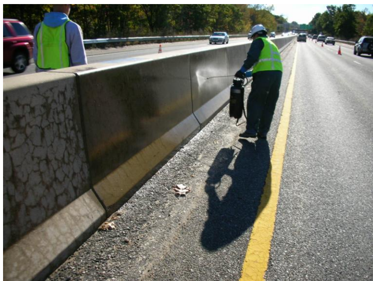
Figure 6. Photograph showing topical application of 40 percent-Silane Solution (solvent-based) to ASR-affected highway barrier in Massachusetts.
