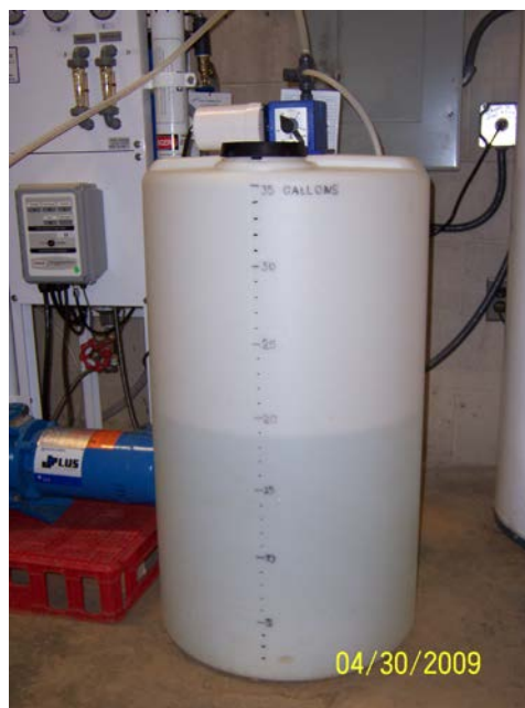
Figure 4-12. Chlorine Addition System at CES
