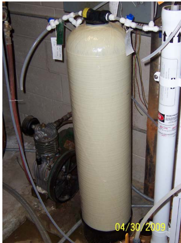
Figure 4-10. Calcite Filter
