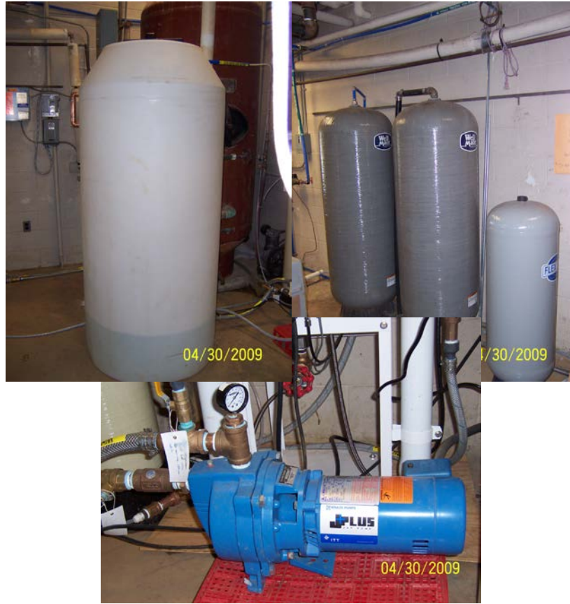
Figure 4-11. Atmospheric Storage Tank (top left), Re-Pressurization Pump (bottom), and Pressure Tank and Retention Tanks (top right)
