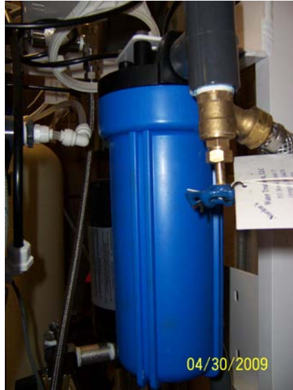
Figure 4-7. Sediment Filter
