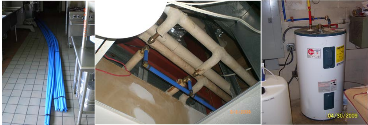
Figure 4-3. Installation of Dual Plumbing System Using PEX Piping (from left to right: prior to Installation, through Ceilings, and to a Hot Water Tank)
