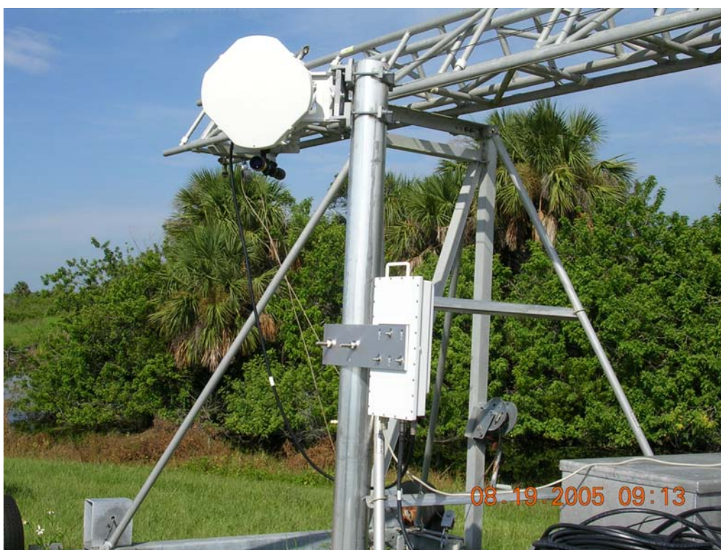
Figure 3-6 Pole Mount with AirPair 100 Modem, Radio, and Antenna
