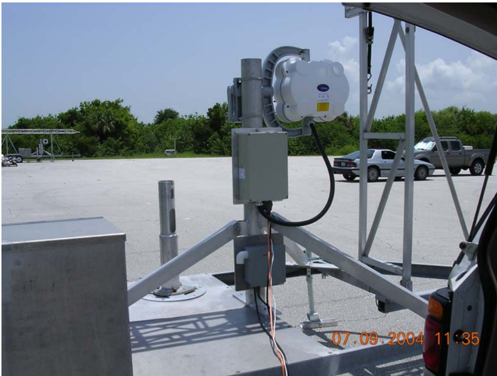
Figure 2-19 Pole Mount with OTU, Connection Box & Power Supply Box
