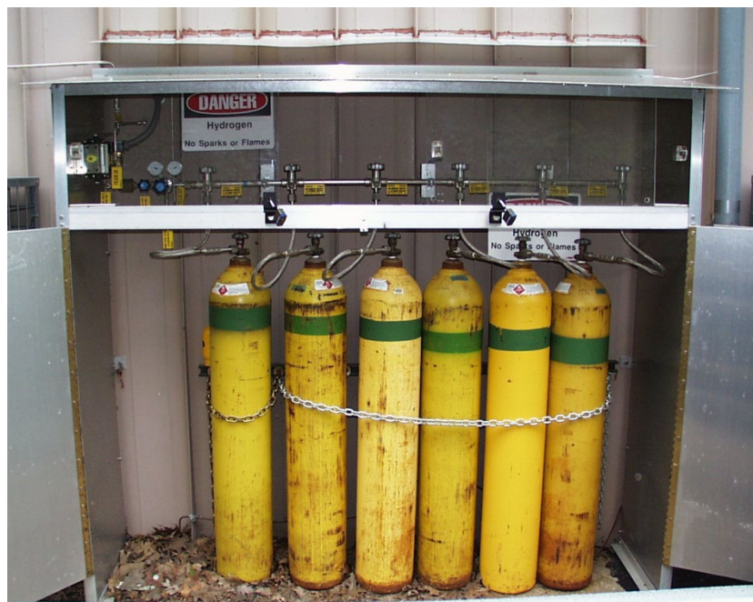
Figure 10.—Close-up view of the hydrogen gas supply manifold.
