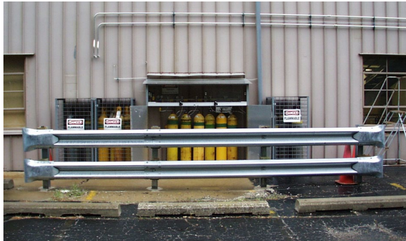
Figure 9.—Hydrogen gas supply manifold and cylinder storage.
