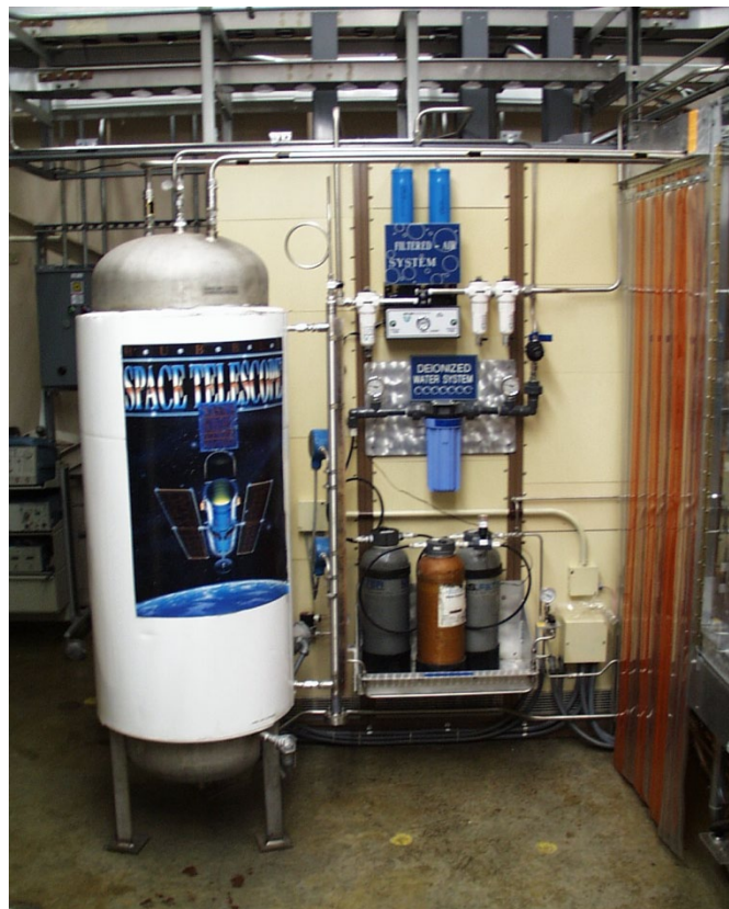
Figure 11.—Hardware used for filtering/humidifying the supply air and deionizing tap water as the supplied cooling media.
