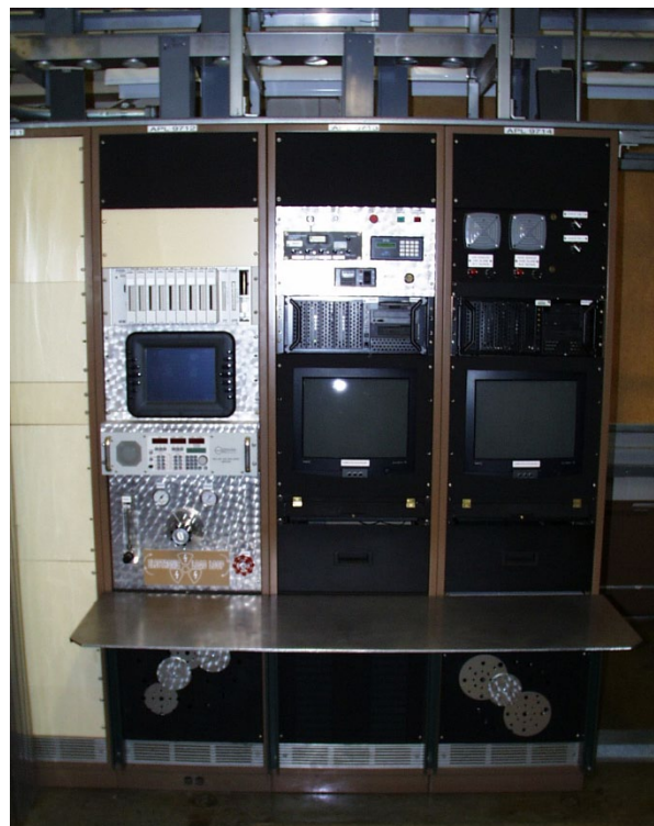
Figure 14.—PLC, data acquisition, ventilation and ancillary system controls.
