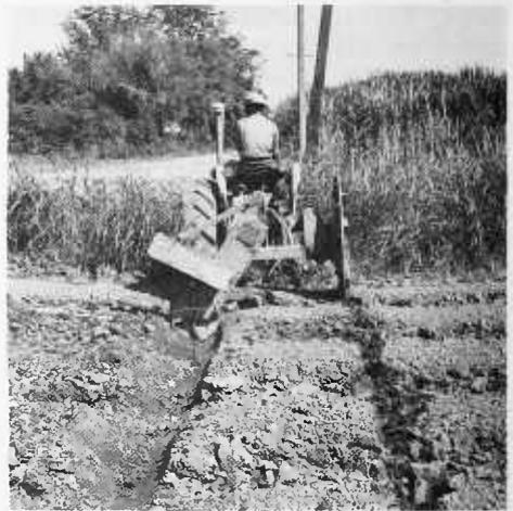
FIGURE 13.—Opening a quarter drain with a tractor plow.
