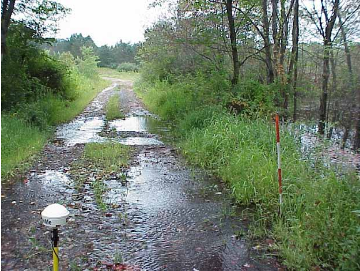
Figure 14. Backwater flooding on a tank trail resulting from a beaver dam plugging the culvert below an existing tank trail.
