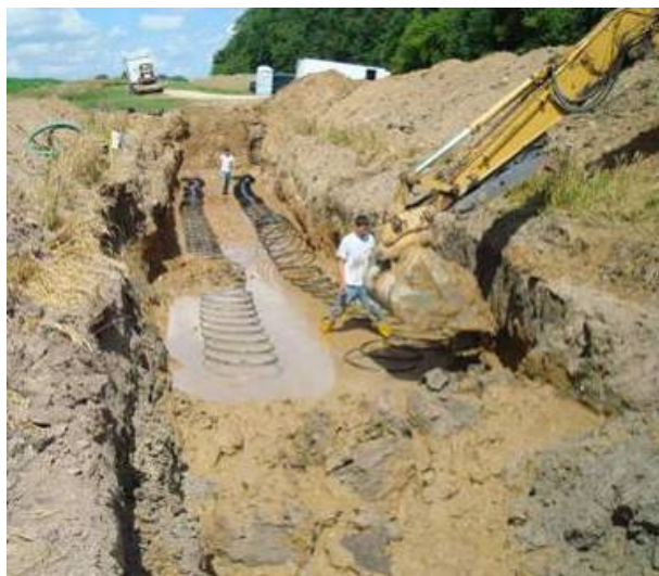
Figure 9 Installation of ground loop at Stoughton residence (image courtesy of WPPI Energy)
