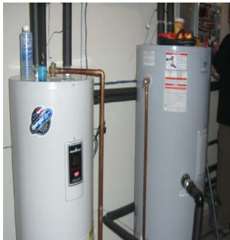
Figure 15. Buffer tank and storage tank in Stoughton home
