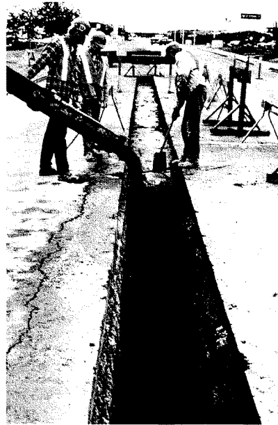
Fig. 2.2—Backfilling utility cut with CLSM.
