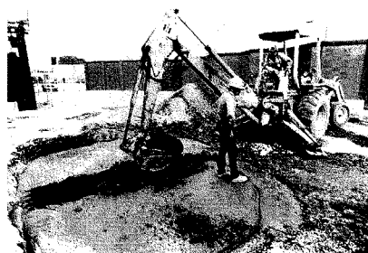
Fig. 4.1—Excavating CLSM with backhoe.
