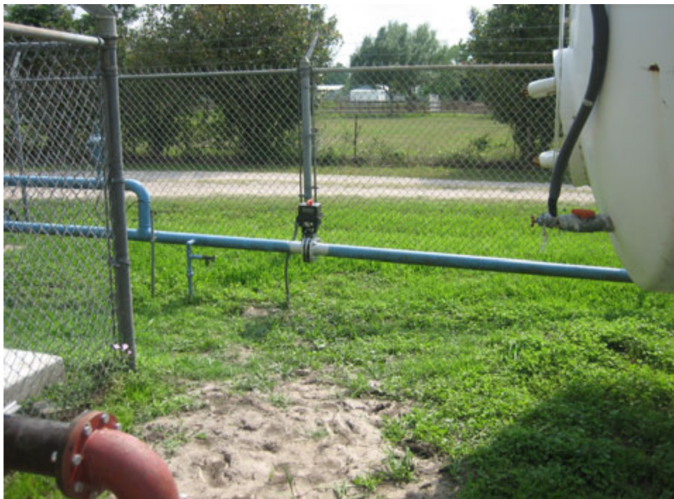
Figure 4-9. Valve MB-127 to Supply Additional Treated Water from Hydropneumatic Tank During Backwash
