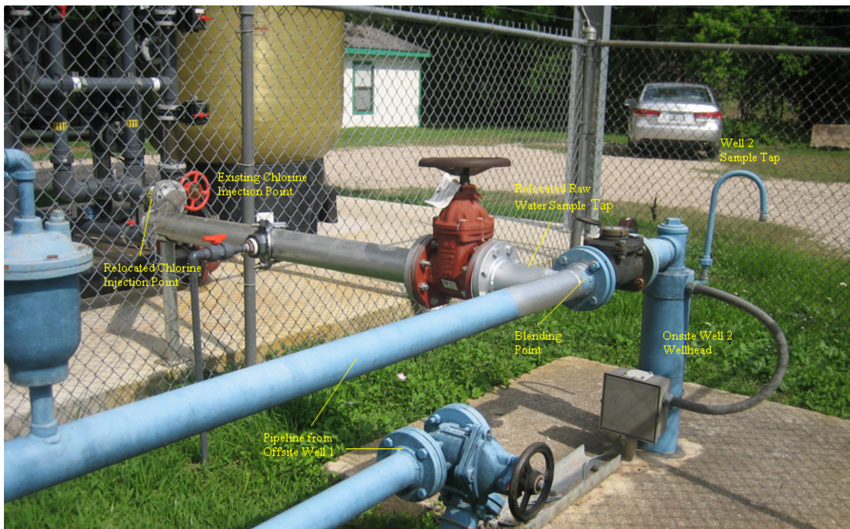
Figure 4-12. Piping, Sample Taps, and Chlorine Injection Point Prior to Treatment System
