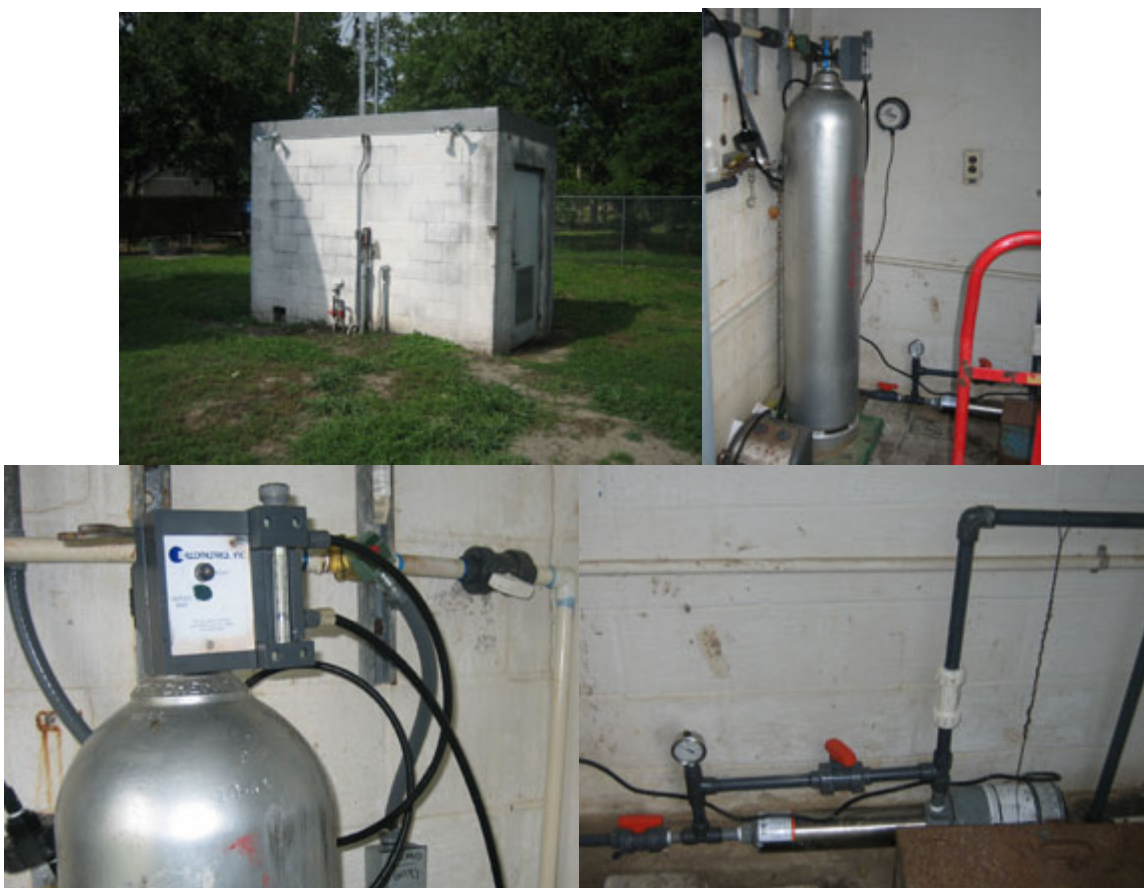
Figure 4-7. Gas Chlorination System (Clockwise from the Top: Shed Housing Gas Chlorination System, Gas Cylinder, Chlorine Ejector, and Chlorinator Unit)
