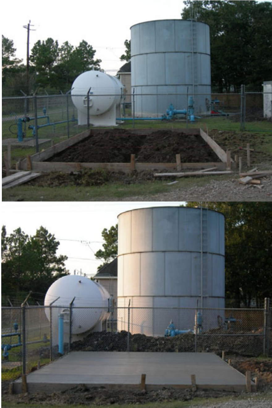
Figure 4-11. Construction of Concrete Pad with Storage Tank and Hydropneumatic Tank (in Background)
