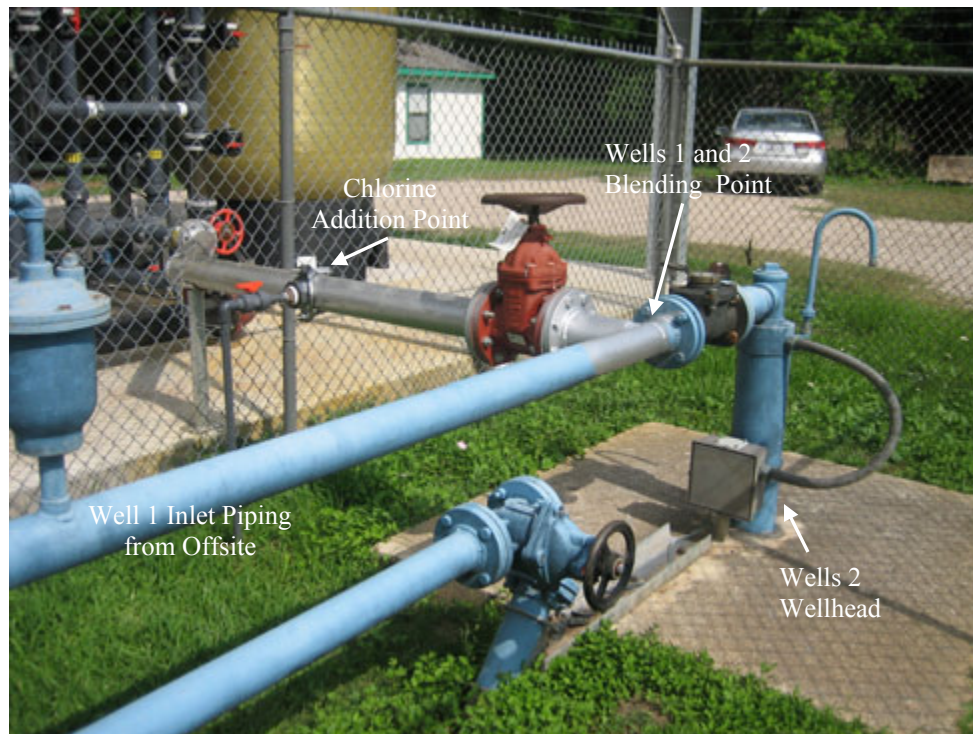
Figure 4-1. Chlorine Addition Point and Wells 1 and 2 Blending Point (Pre-existing)
