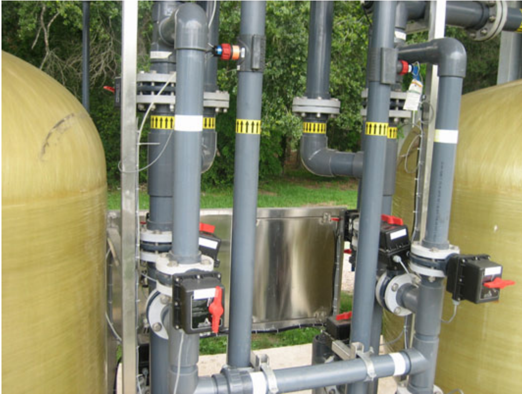
Figure 4-8. APU-30S System Valve Tree and Piping Configuration
