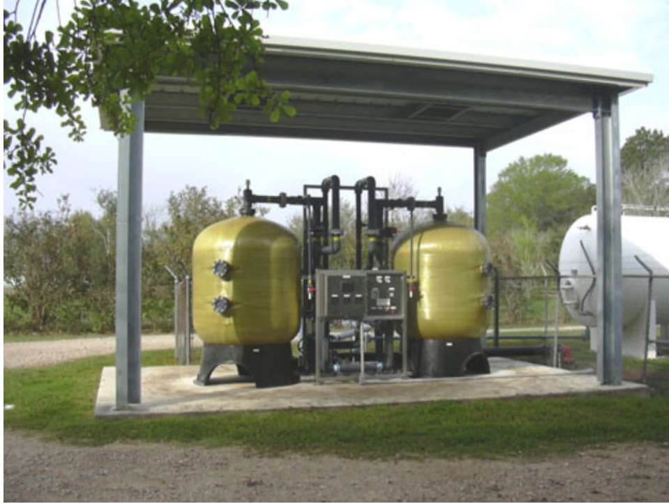
Figure 4-5. APU-30S Arsenic Removal System
