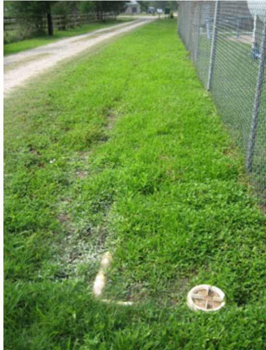
Figure 4-10. Small Ditch for Backwash Wastewater
