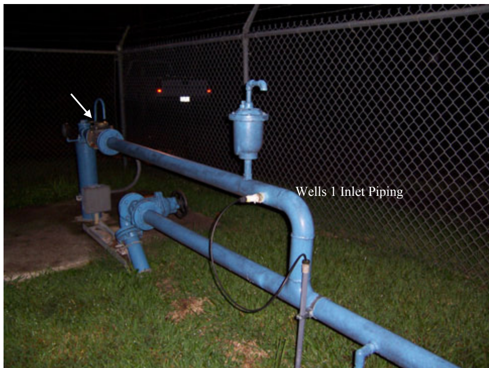
Figure 4-3. Pre-existing Polyphosphate Addition Point
