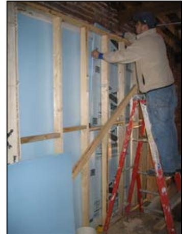
**Figure 21. Slide insulation in behind existing stud wall**
