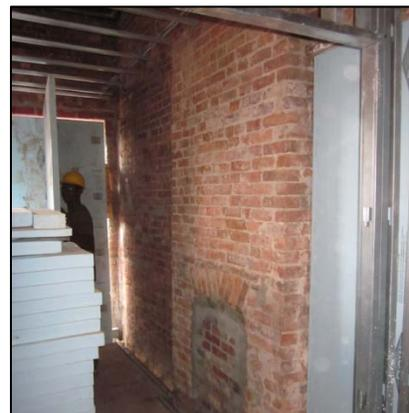
**Figure 9. Example of wall ready for insulation**
