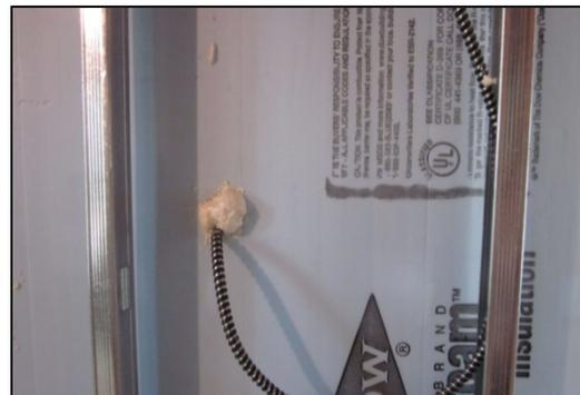
Figure 15. Seal all penetrations through the rigid board with foam
