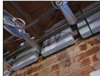
Figure 18. Rigid insulation extends past the sub-floor when installed from above
