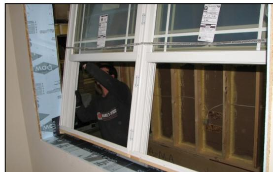
Figure 19. Installing a window after installing insulation and flashing. XPS insulation was placed between the window buck and the interior jamb extension (not yet installed) of this modular home.
