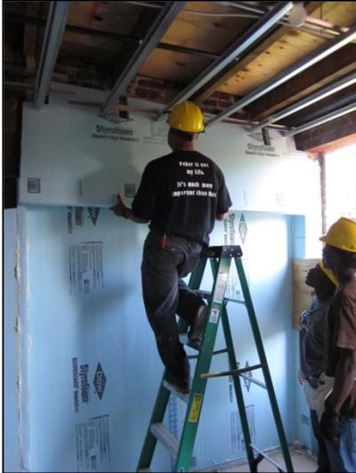
Figure 16. Install insulation from below
