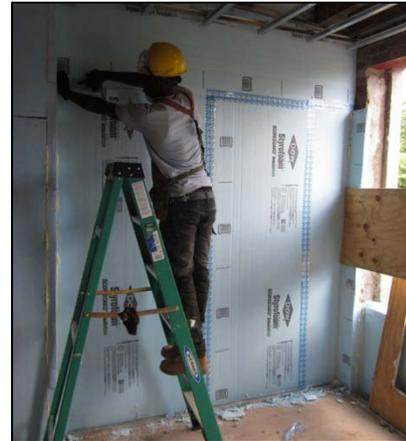
Figure 13. Tape over seams less than 1/8" wide
