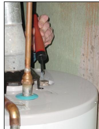
**Figure 22. Spillage testing of an atmospherically vented, natural gas water heater**
