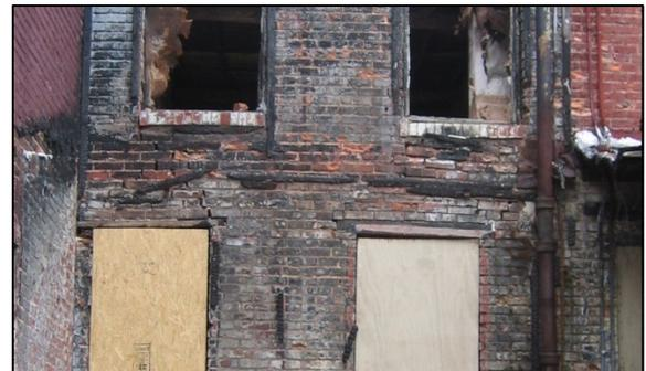
Figure 7. Heavily deteriorated brick wall
