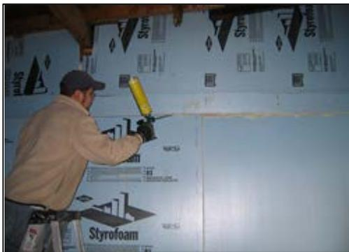
Figure 14. Use foam to seal all seams greater than 1/8" wide
