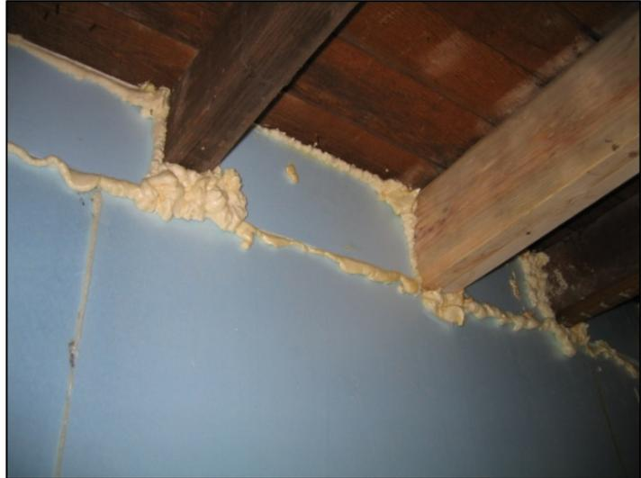
Figure 17. Seal all seams with low-expanding foam
