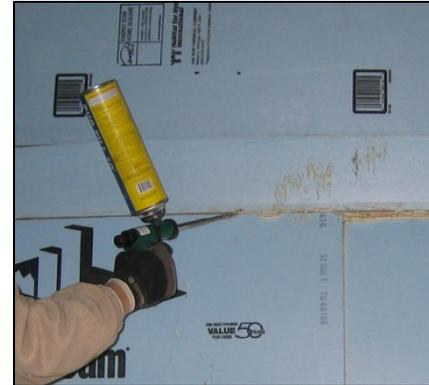
**Figure 6. Low-expanding foam sealant and applicator**
