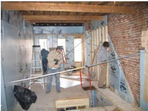
**Figure 11. Bracing insulation on opposite walls**
