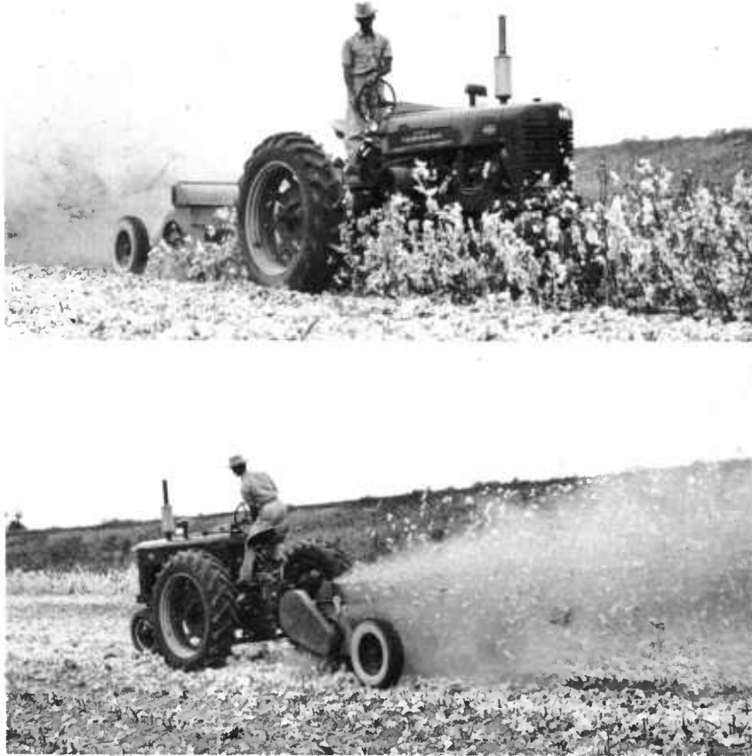
Figure 13.—Stalk shredding with flail shredder ( top ) and machine lifting bolls from ground and shredding them ( bottom ). PN-4430
