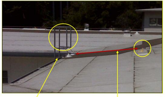
Figure 6. Rooftop of Building 161 – Rooftop Access and Distance to Fall Restraint System
