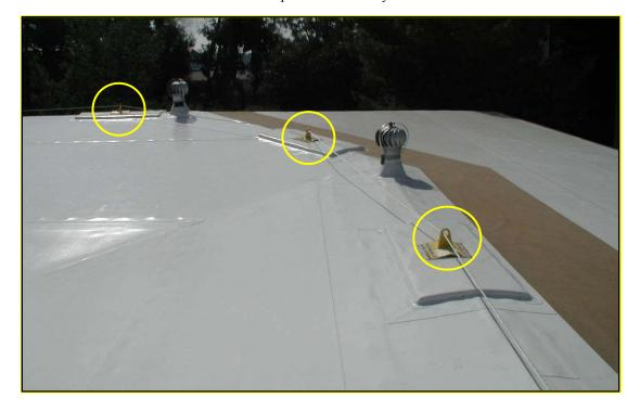
Figure 5. Rooftop of Building 156 Rooftop Fall Restraint System
