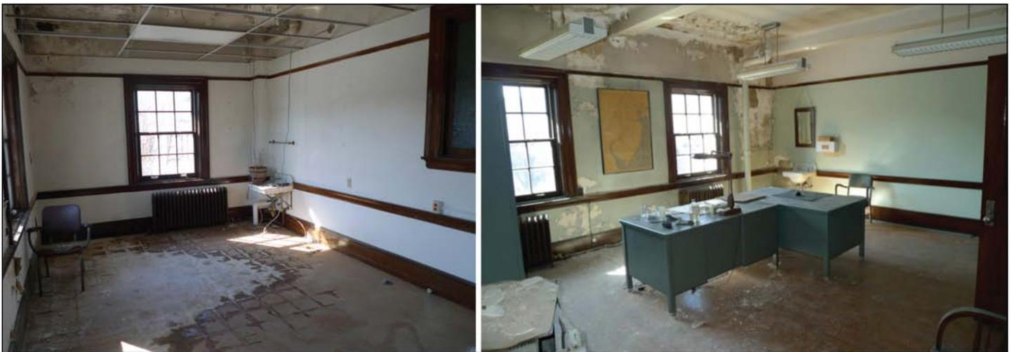
Upstairs offices in the Easton Main Post Office with walls, ceilings and floors damaged by water.
