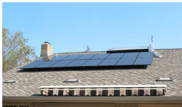
(b) The 2.3 kW PV array and the ISC SWH. Also shown is the weather station installed by NREL. NREL/PIX 19615, Credit: Lieko Earle
