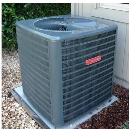
(b) High efficiency SEER 16, HSPF 9.75 heat pump (condenser unit) Credit: Judy Lew-Loose, SMUD
