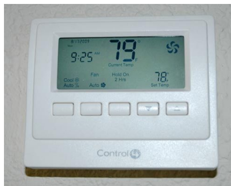
Figure 20. Control4 thermostat can be controlled manually or remotely
