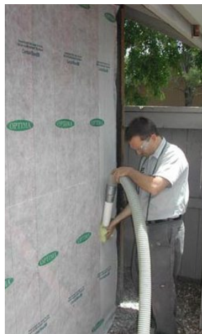
(a) Dense pack blown-in cellulose being installed in the west wall. Credit: Judy Lew-Loose, SMUD.
