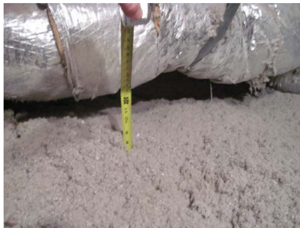
(b) Blown-in cellulose in the attic covered fiberglass batts. NREL/PIX 19612, Credit: Lieko Earle
