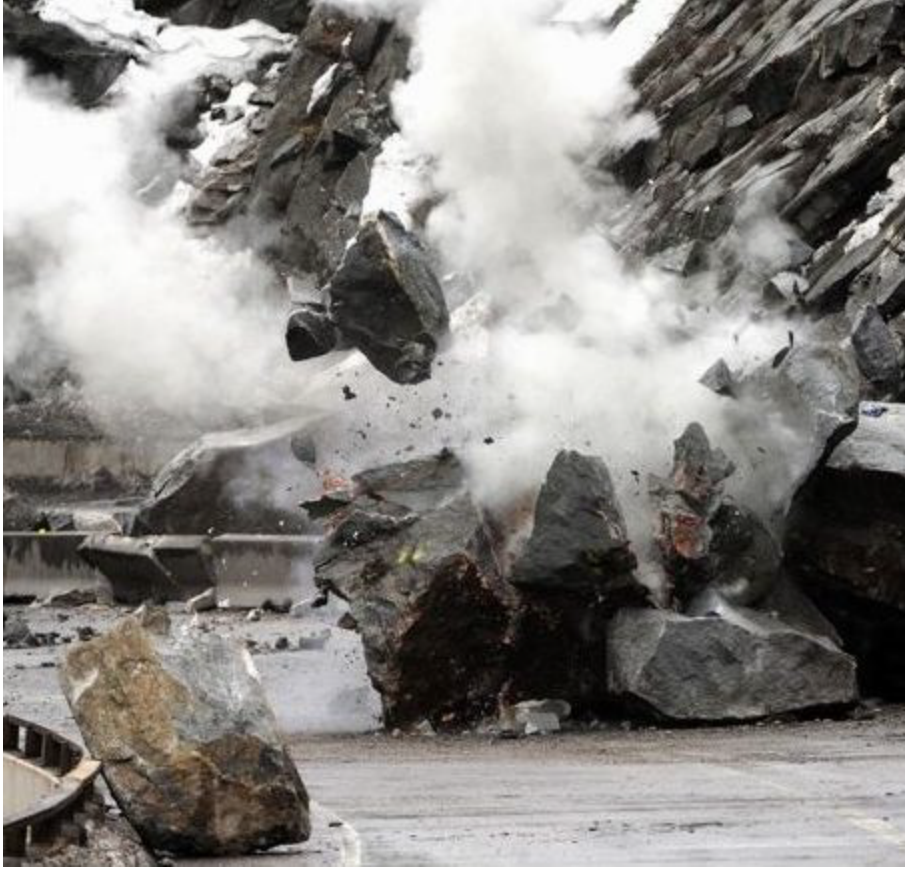
Figure 5. Rock-blasting by Colorado Department of Transportation (CDOT) after the March, 2010, Glenwood Canyon rockfall, on Interstate-70. These rocks were removed because they were precariously poised above the rockfall area, could endanger workers repairing the highway, and could possibly be a threat to the highway in the near future. Photograph by CDOT.
