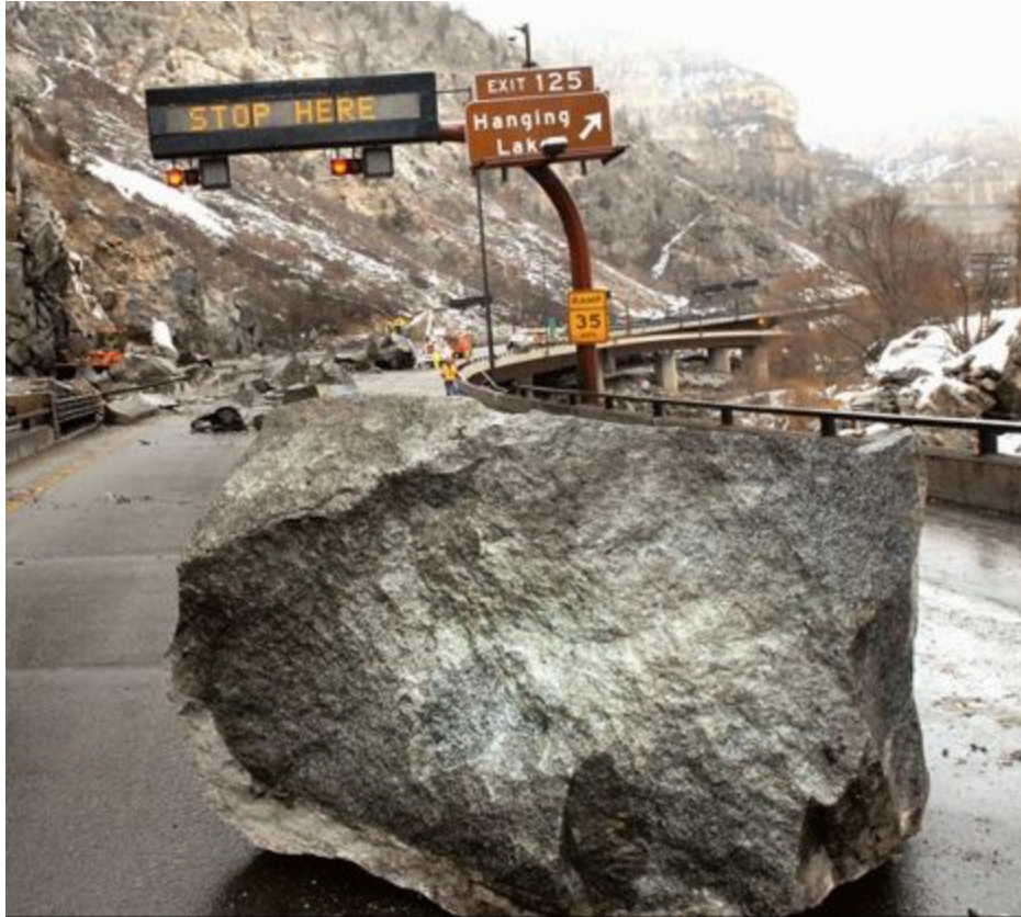
Figure 3. Interstate-70 in Glenwood Canyon, Colo. The March 8, 2010, rock slide closed the highway and damaged this elevated portion of Interstate-70. Photograph by Colorado Department of Transportation.
