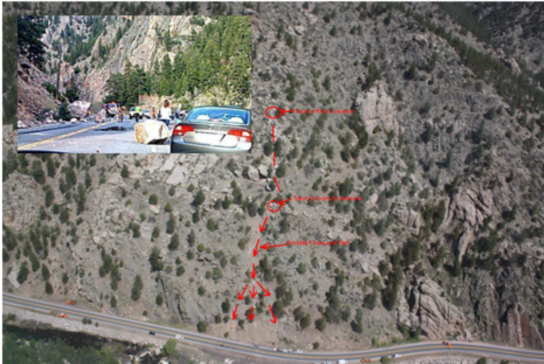
Figure 7. Photograph of the source area of the May 21, 2010, rockfall that impacted Highway 34 near Estes Park, Colo. Inset shows a road-level photograph of the area on the highway where rocks fell. Photograph and graphics courtesy of Tyler Ortiz, Colorado Department of Transportation.
