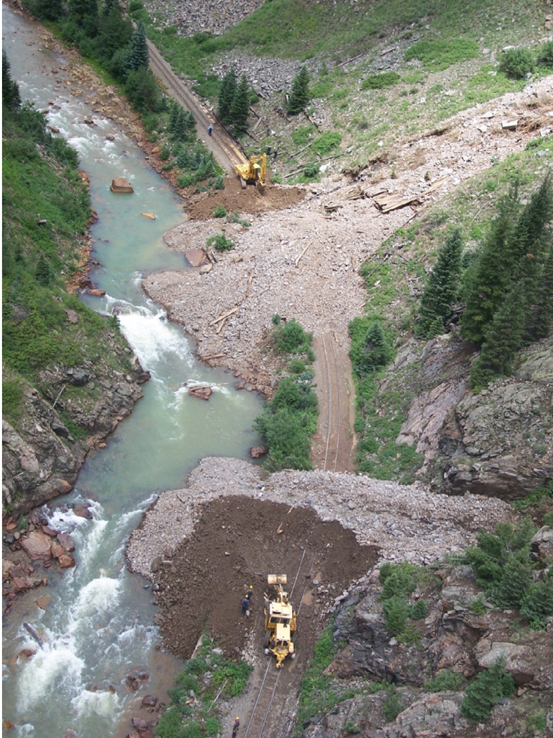
Figure 16. A close-up aerial view of the two debris flows that blocked the Durango Silverton Narrow Gauge Railroad track in July, 2010. Cleanup was performed by railroad crews. Photograph courtesy of Tall Timber Resort/Soaring Tree Top Adventures.
