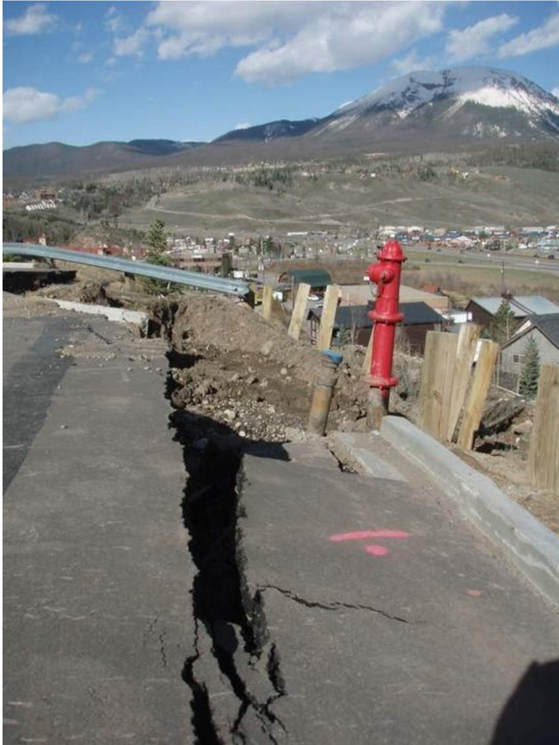
Figure 23. Slumping roadway above a retaining wall near Dillon Valley Reservoir. Officials are trying to determine what caused the retaining wall to fail after a water main broke nearby. Photograph by Lake Dillon Fire-Rescue.
