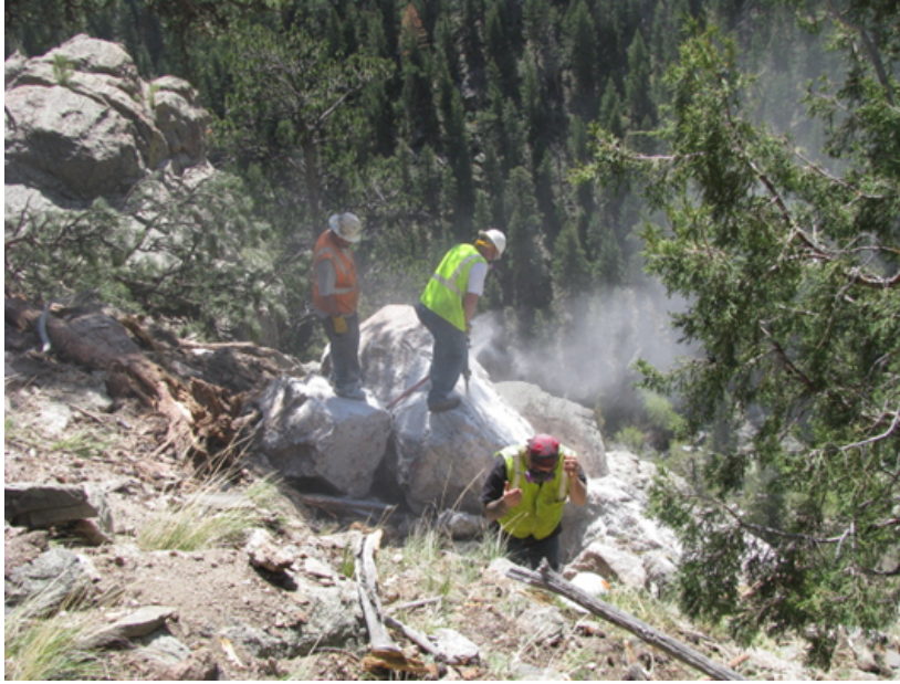
Figure 8. Colorado Department of Transportation (CDOT) crews breaking up rocks above the closed Highway 34 after the rockfall event of May 21, 2010, near Estes Park, Colo. The rock was brought down and hauled away to mitigate the rockfall hazard. Photograph courtesy of Tyler Ortiz, CDOT.
