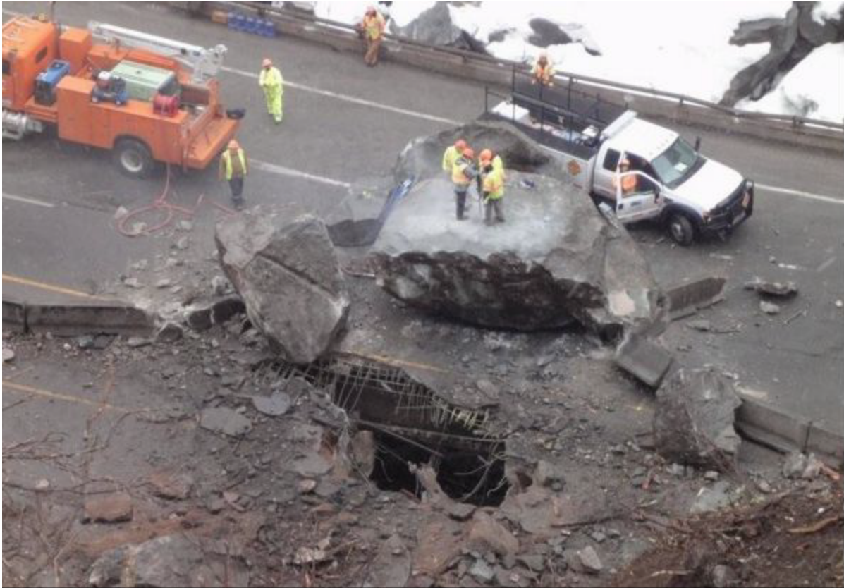
Figure 4. Photo showing an overview of the 2010 Glenwood Canyon, Colo., rockfall showing damage to the road deck on the elevated portion of Interstate-70. Photograph by Colorado Department of Transportation.
