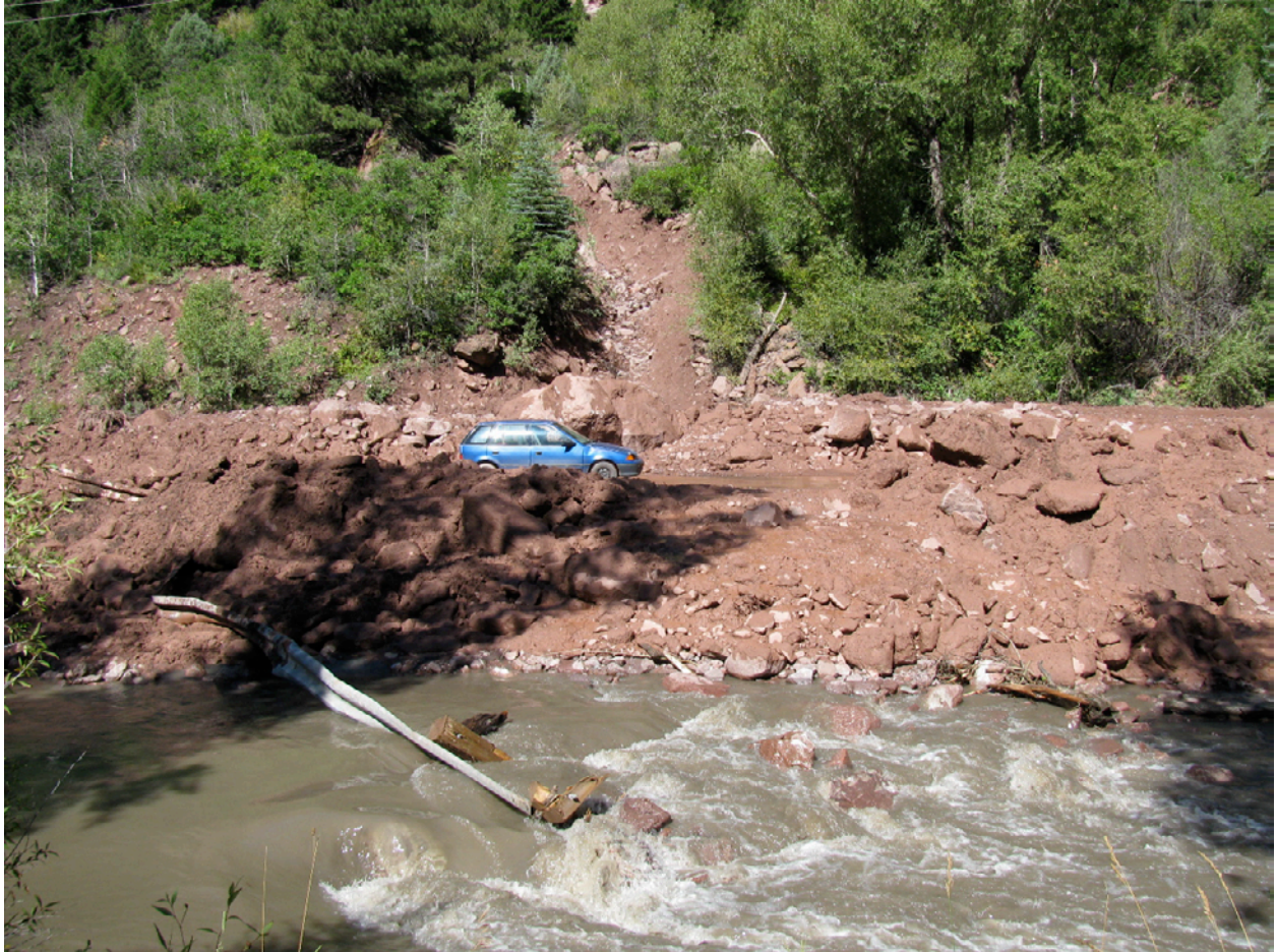
Figure 12. August 19, 2010. Highway 133 was closed at Redstone, Colo., for several hours, but crews were able to reopen one lane. There were six drainages where mud crossed Highway 133, taking out 100 feet (33.3 meters) of guardrail. The Crystal River (which flows parallel to Highway 133) is shown in the foreground. Photograph by Sue McEvoy.
