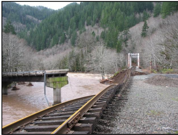
A flood on December 3, 2007, undermined bridge piers and railroad tracks adjacent to the Salmonberry River near its confluence with the Nehalem River (Oregon Department of Forestry).
