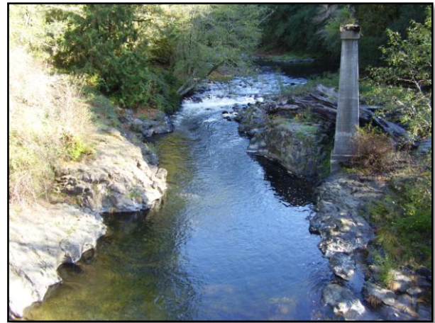
Bridge pier blocking large wood on the North Fork Trask River near its confluence with the South Fork Trask River.
