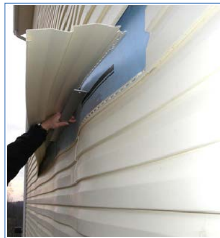
Figure 4. Wall with buckled OSB panels (siding removed exposing the weather-resistant barrier)
