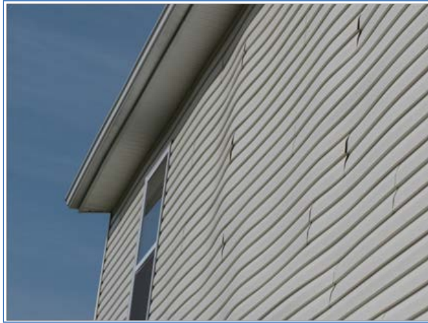
Figure 1. Wavy lap siding resulting from buckled OSB panels on the rear wall of a house
