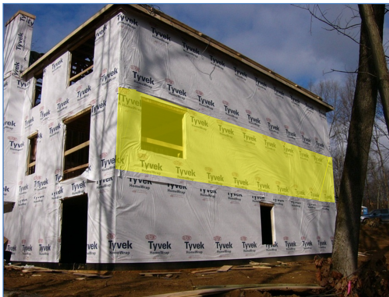
Figure 14. Jobsite 2 east wall (test wall highlighted), three stories framed
