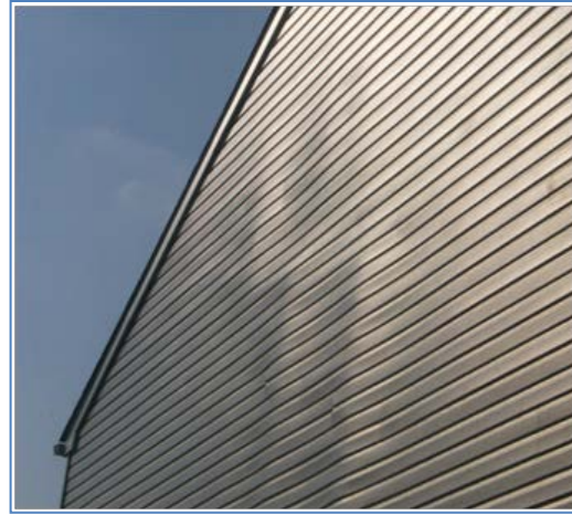
Figure 2. Wavy siding resulting from buckled OSB panels on a side wall of a house
