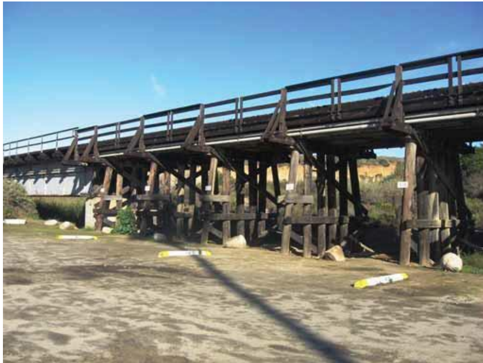
a) View of Green Beach Bridge South Trestle Pile Bents 1 to 5
