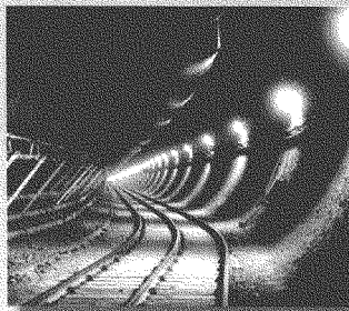
The main tunnel under Yucca Mountain, showing ventilation pipes and train tracks.
