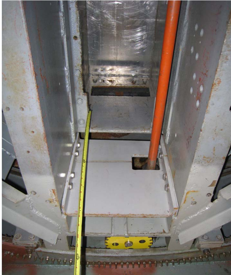
Figure 7.4-2. Turntable Cruciform Base and Support Tube
