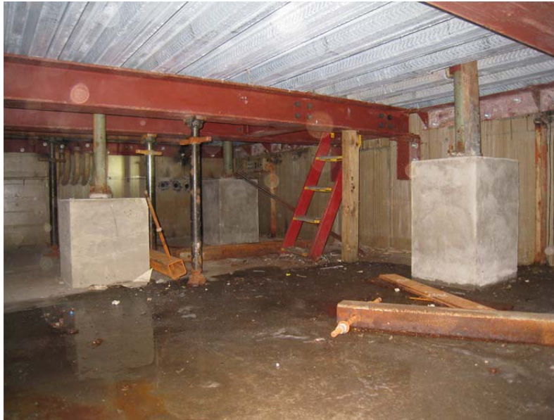
Figure 7.4-1. Load Path Termination in Tunnel. The photo shows the former cylindrical balance columns now mounted to blocks of concrete. This is directly beneath the floor area that is below the test section/turntable/balance system.
