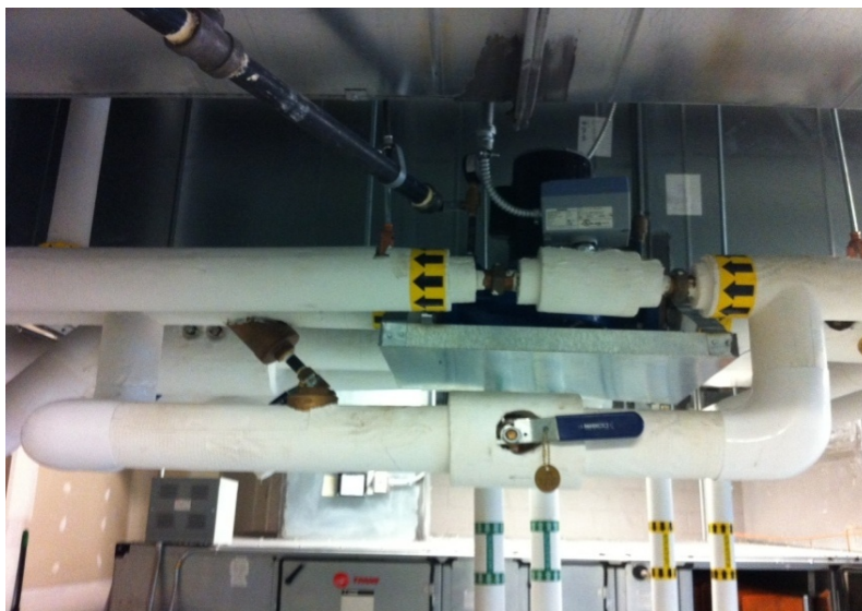
Figure 23 – Two Way Control Valve with Bypass Image Credit: Jesse Dean (NREL)
