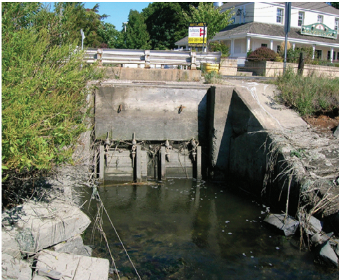
Figure 5. The tide gate in closed position (left) and the bridge constriction (right) on Sybil Creek, Connecticut.
