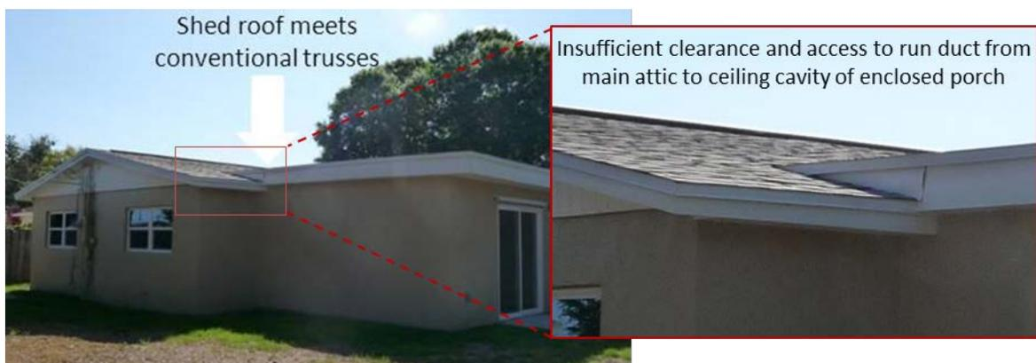
**Figure 9. Intersection of shed or flat roof with conventional trusses (left) at enclosed porches creates a very shallow connection (right) to the main attic. Limits room for routing ductwork.**
