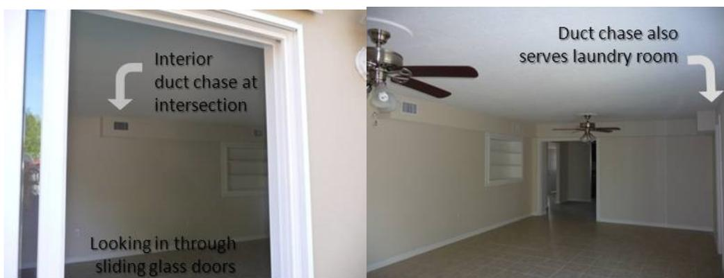
**Figure 11. Interior duct chase eliminates need for panned ceiling cavity**
