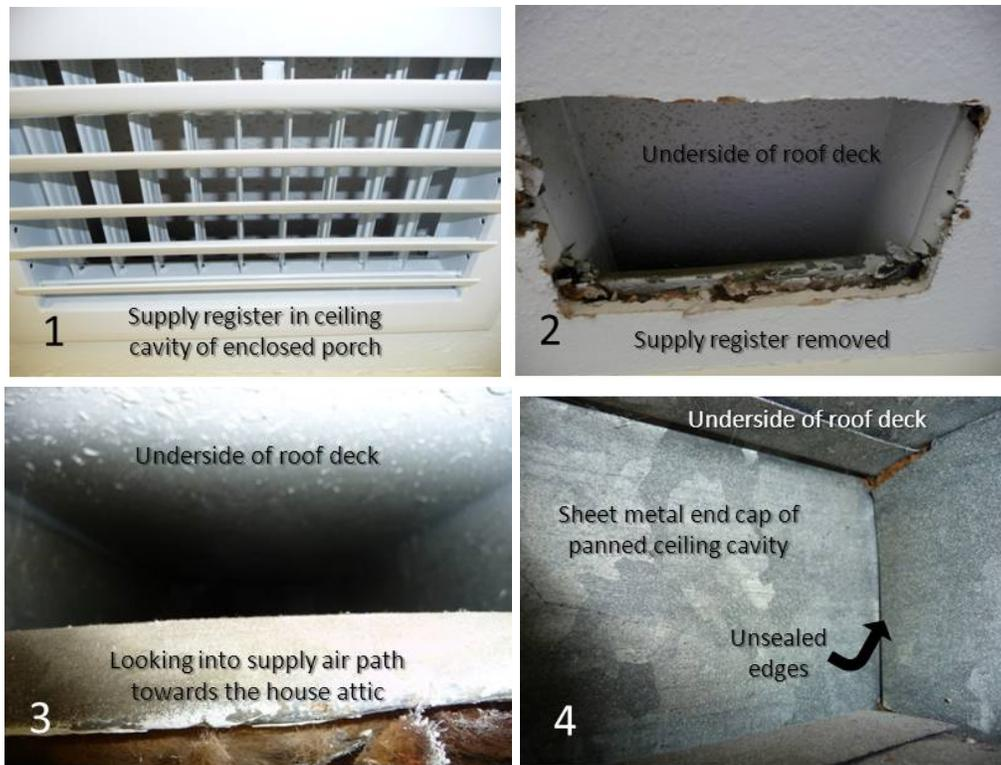
**Figure 10. Panned ceiling joist details common to enclosed porches**
