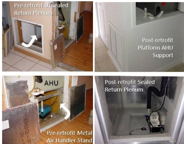
**Figure 5. Pre-retrofit metal AHU stand with no dedicated return air path (left); post-retrofit platform AHU support with dedicated, mastic sealed return air path (right)**
