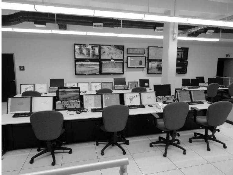
Figure 3.—The modernized control room for B-2. Graphical user interfaces (GUI) for the programmable logic control (PLC) based system are visible in the foreground. Along the back wall, video monitors display test site camera images.
