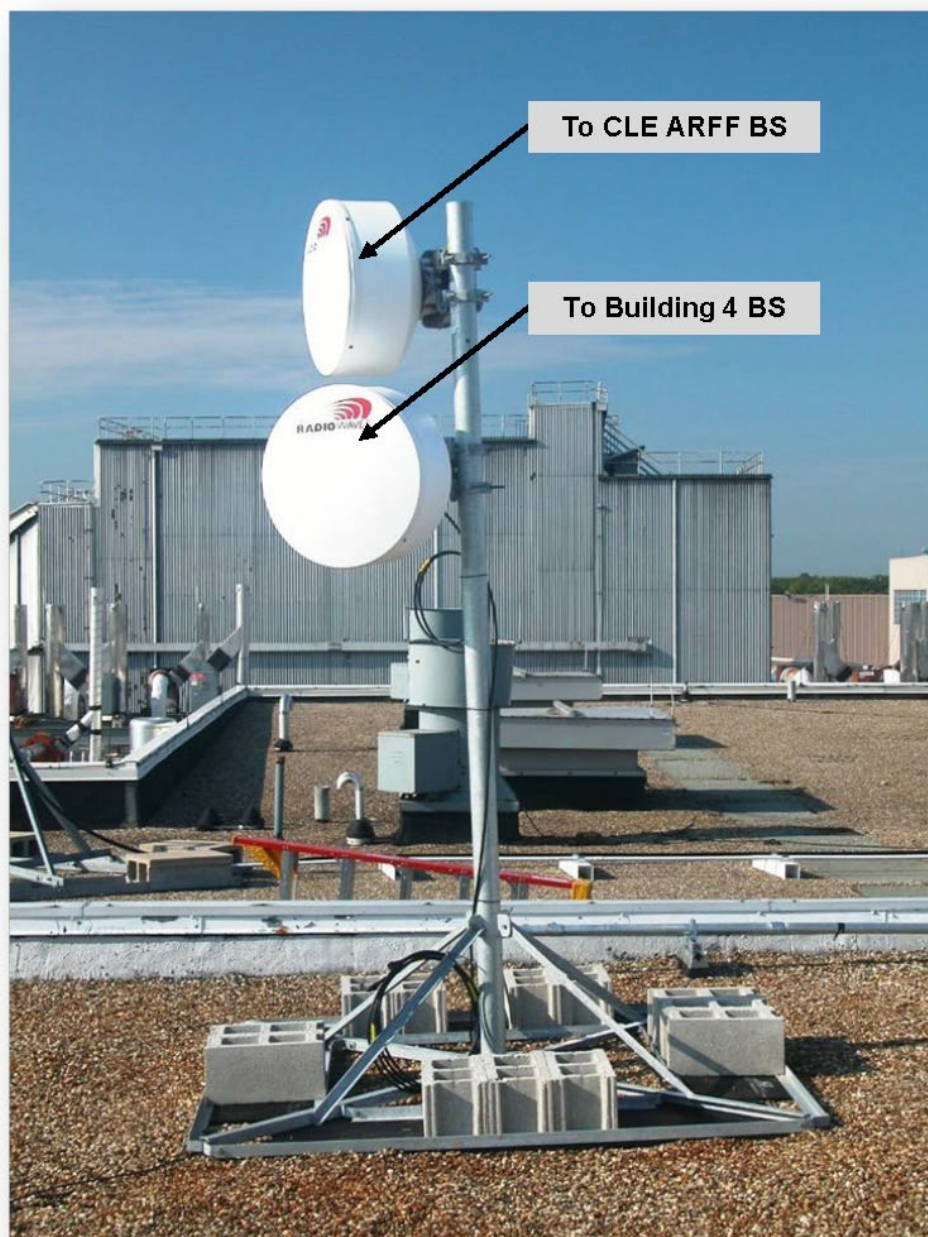
Figure 40.—11-GHz backhaul radio outdoor units at Glenn Building 110 with links to Glenn Building 4 base station (BS) and to Cleveland Hopkins International Airport's (CLE) Airport Rescue and Firefighting (ARFF) building.
