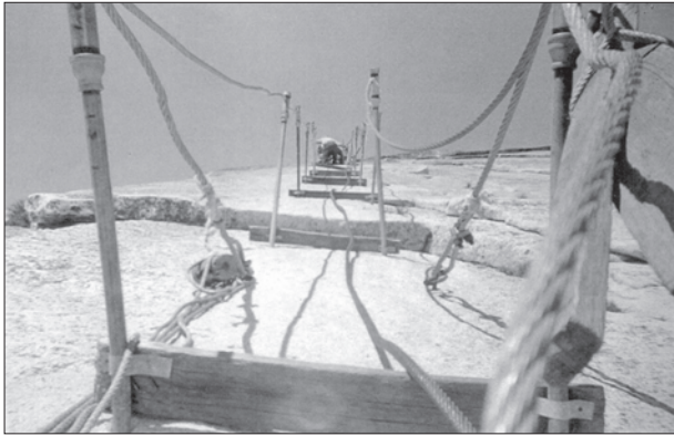
Figure 30. Ascent of Half Dome at Yosemite National Park by steel pipe and cables installed by the CCC in 1939. (National Archives; NARA MD 79G-17C-4. May 1939)
