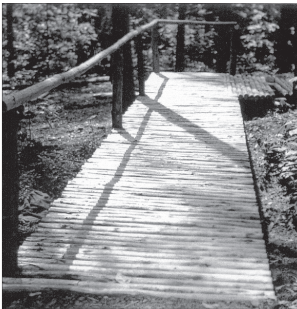
Figure 23. Historic photograph of corduroy bridge constructed by the CCC in Shenandoah National Park in Virginia. (National Archives; NARA MD, 79-42, VA, Box 32)
