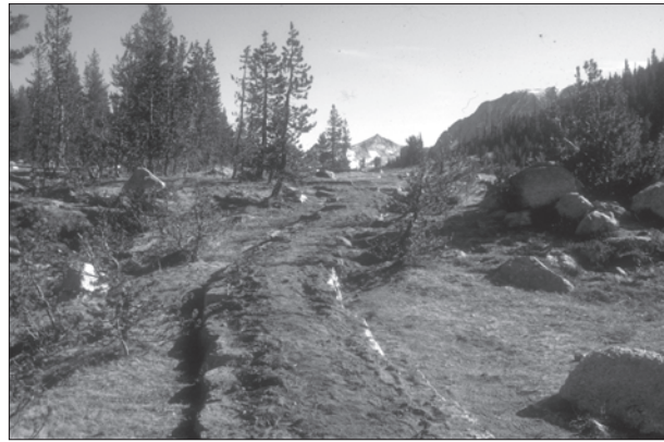
Figure 37. This stone-lined causeway with crowned tread material was constructed in 1985 through Rafferty Meadow in Yosemite NP to repair eroded alpine area. Because the trail is located in a designated Wilderness area, materials were imported by mule. (NPS, Steve Griswold)
