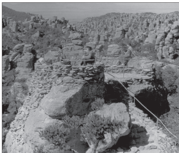
Figure 9. The lookout platform at Massai Point, Chiricahua National Monument, completed by the CCC in 1935, is an example of highly crafted stone steps, stone walls, and ironwork constructed to harmonize with the natural scenery. (NPS Historic Photo Collection, Harpers Ferry Center)
