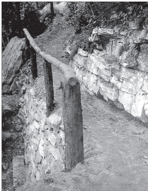
Figure 14. Historic photograph of horse trail, retaining walls, and guard rail built by the CCC in 1935 for a trail south of Sunset Rock in Chickamauga & Chattanooga National Military Park, Georgia. (National Archives; NARA MD, 79-42, GA, Box 14)
