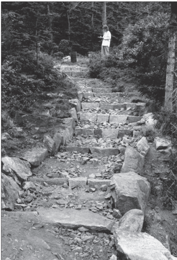
Figure 39. A section of checks installed to repair a gullied trail shown during and after completion on the Ocean Path at Acadia National Park. (NPS, Olmsted Center for Landscape Preservation)
