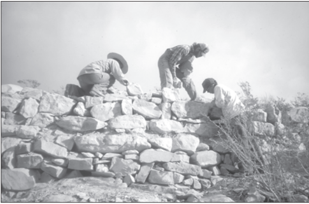
Figure 32. Nearly complete rebuilt wall at Big Bend National Park. To preserve the rough appearance, stones were placed with varied orientations. To improve stability, backfill was carefully laid. The wall was topped with large coping stones and the load was transferred down through the semi-laid backfill. (NPS, Steve Griswold)
