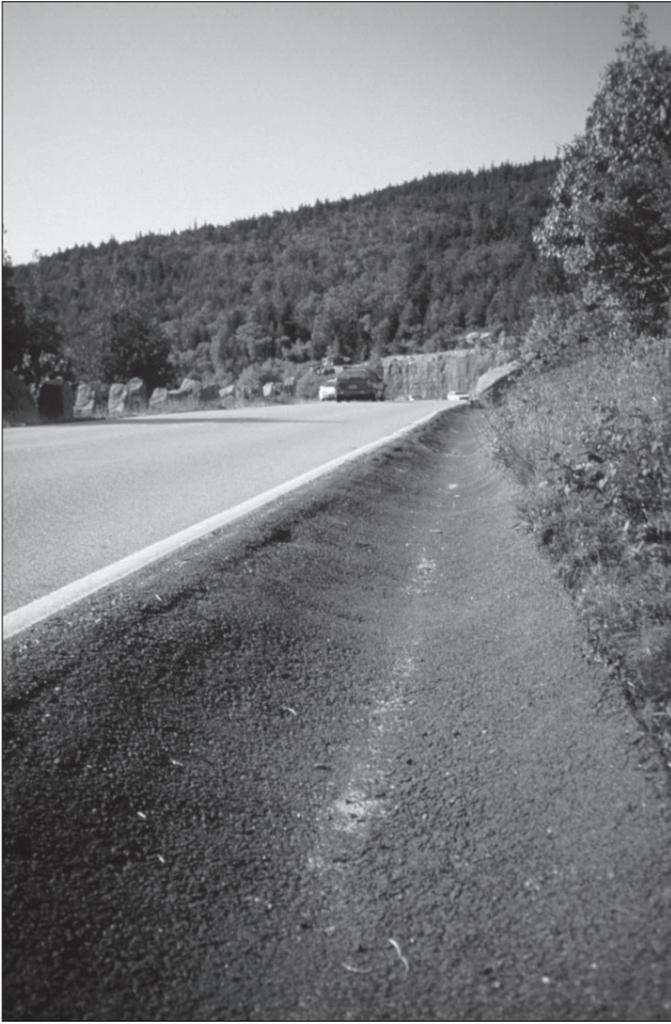
Figure 23. Many historic gutters have been overlain with bituminous concrete to ease maintenance and repair; such inappropriate treatments should be reversed whenever possible. (Foulds 1993)
