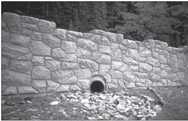
Figure 27. Simulated stone retaining wall with integral culvert and crenellations: this treatment is best restricted to areas where visitors do not come close enough to discern the artificial nature of the materials, Yellowstone National Park. (Davis 1996)
