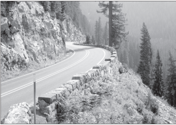
Figure 6. Classic crenellated stone guardwall, West Side Highway, Mount Rainier National Park. (Historic American Engineering Record [HAER] 1993)
