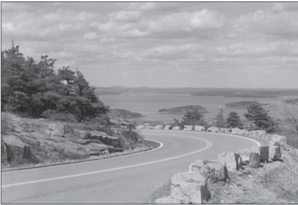
Figure 28. Historic stone safety barriers have functioned successfully in the low-speed, low-volume context of most park roads; Cadillac Mountain Road, Acadia National Park. (HAER 1995)
