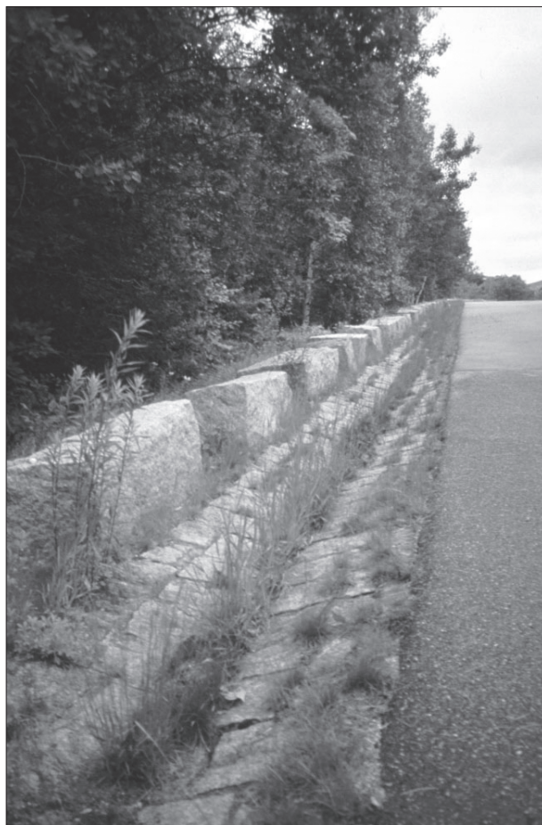
Figure 22. Attentive maintenance is necessary to ensure that historic drainage features such as these stone-lined gutters in Acadia National Park do not become obstructed by vegetation, siltation or other natural processes. (Foulds 1993)
