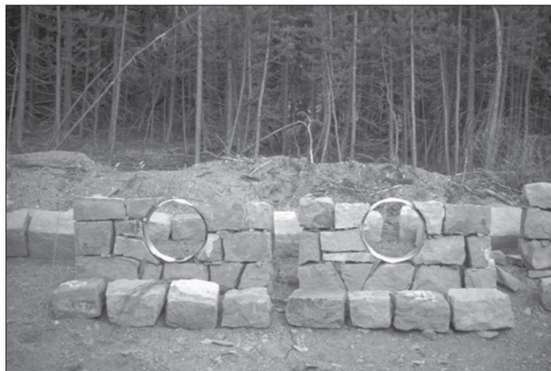
Figure 25. Modern pre-cut stone headwall awaiting installation on road rehabilitation project, Yellowstone National Park. (Davis 1996)
