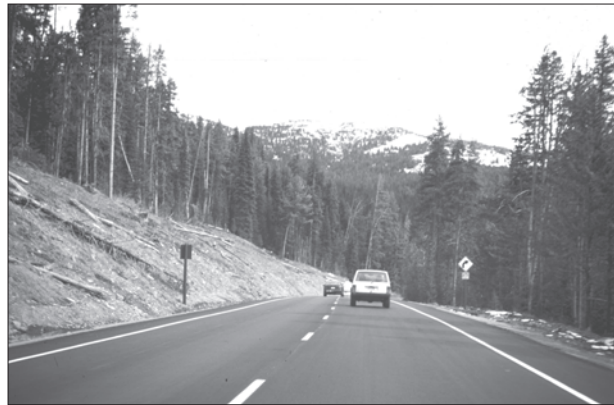
Figure 38. Cutting a broad clear zone can improve safety by providing motorists more room to recover from potential accidents, but this approach markedly alters the motorist's perspective and produces greater separation between visitors and their surroundings, rehabilitation of East Entrance Road, Yellowstone National Park. (Davis 1996)
