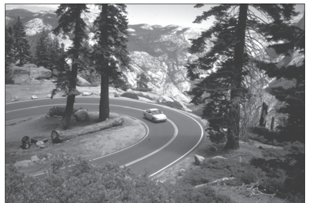
Figure 20. Classic park road with tight curvature calculated to provide thrilling views of natural scenery; changing historic alignment to conform to modern standards not recommended; Glacier Point Road, Yosemite National Park. (Davis 2000)
