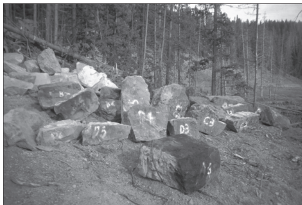
Figure 24. Historic stone culvert headwall salvaged and numbered for reassembly after road-widening is completed, Yellowstone National Park. (Davis 1996)
