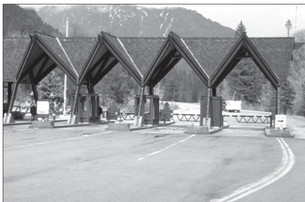
Figure 34. Yellowstone's 1966 East Entrance Station epitomizes Mission 66's creative mingling of modern and rustic styling but is no longer able to accommodate the largest recreational vehicles, which must be routed around the structure. (Davis 1999)
