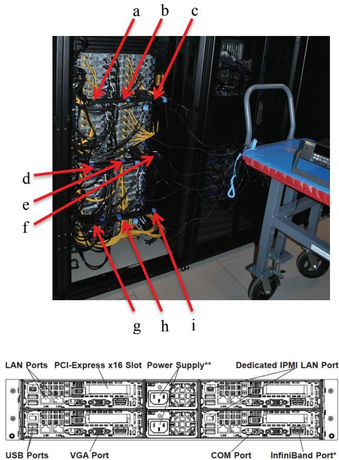
**Figure 10. Temperature sensor arrangement (back of rack) and chassis back view. Images from Super Micro Computer, Inc.**
