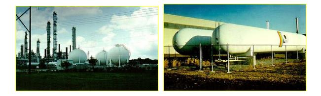
**Ultrahigh-pressure** containers such as tube tanks, pipelines, or cylinders are not common and contain mostly gases and a few liquids. They are usually aboveground and horizontal.
