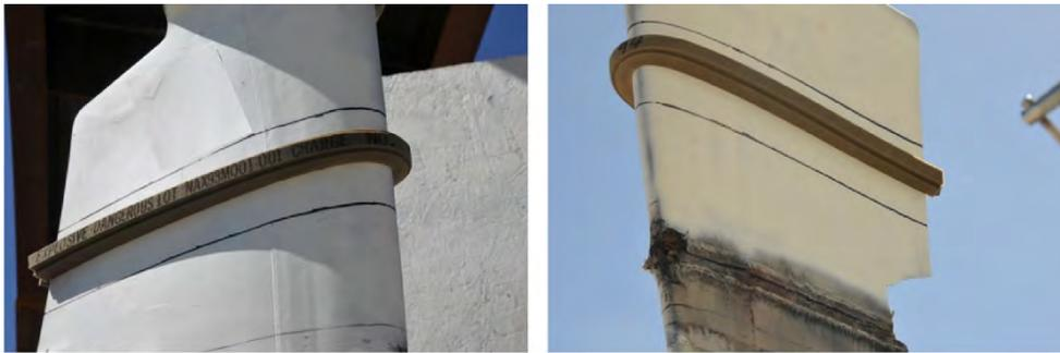
Figure 8.—Blade with shape charge around full circumference.
