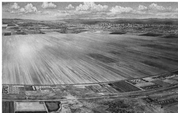
Figure 4. Commercial power receiver, built over farm land, accepting an invisible power beam and feeding clean electric power to a large city and its region
