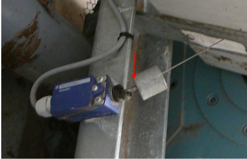
Figure C.7 Broken vibration sensor and deteriorating rubber seal. PIX #17674.
