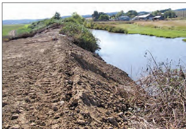
**Figure 7.** Repaired levee separating Wapato Lake and Wapato Creek on the west side of Wapato Lake, Oregon. (Photograph taken by Matt Nussbaumer, City of Hillsboro, September 23, 2008.)
