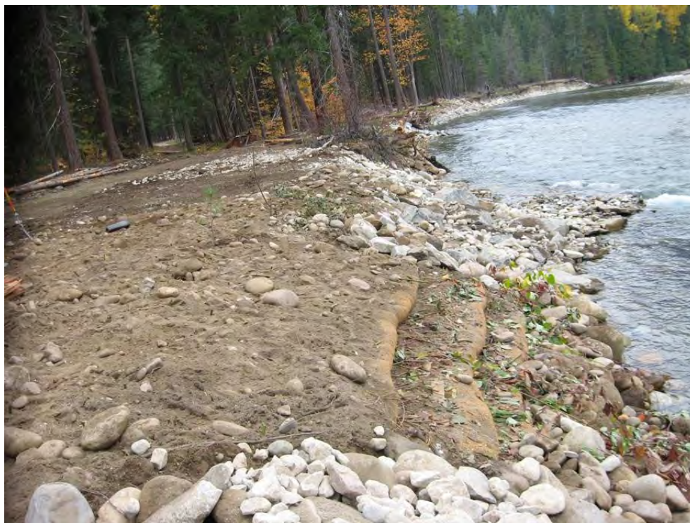
Photo 12 – Rock Barb and Willow Layers (Bioengineering) on Upper Company Creek Road Shortly after Installation
