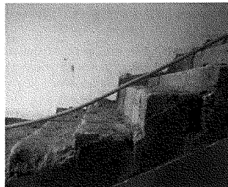
Photo 3 - Stairs of Different Heights and Crumbling at Garm Ser Site
