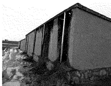
Photo 1 - Exterior View of Building Deterioration Due to Water Penetration
