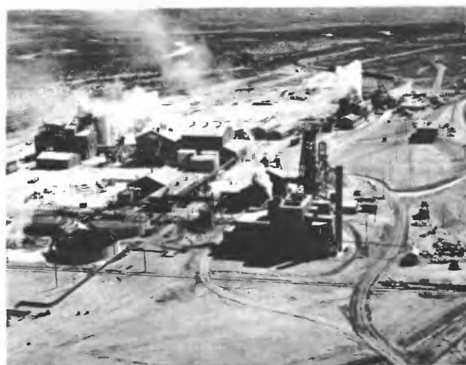
FIGURE 5.—Photograph showing the calcining house, the screen house, and the superstructure of shaft 1 of the Westvaco mine.
