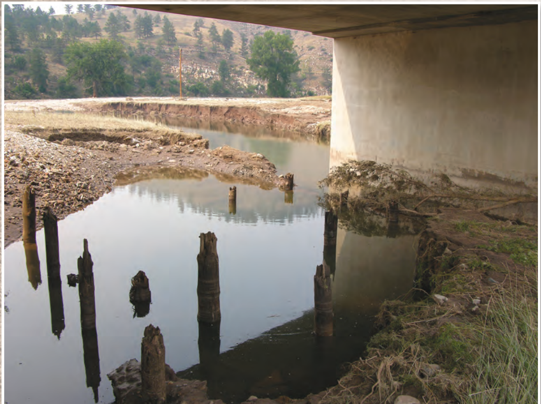
Figure 8. Photographs showing scour from flooding on August 17, 2007, at a bridge site along Highway 40 about 2 to 3 miles west of Hermosa, S. Dak. Photographs by Mark T. Anderson.
