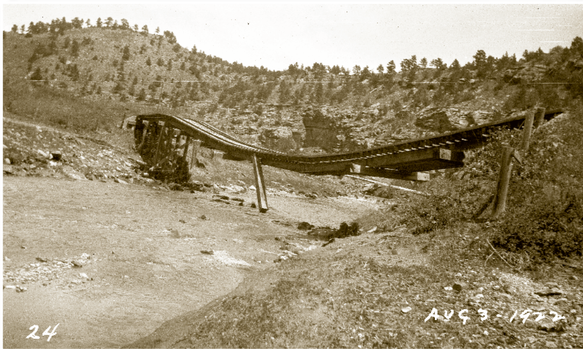
Figure 27. Photograph of damage to a railroad bridge during the August 3, 1922, flood along the Fall River near Hot Springs, S. Dak. (photograph courtesy of Fall River County Historical Society).
