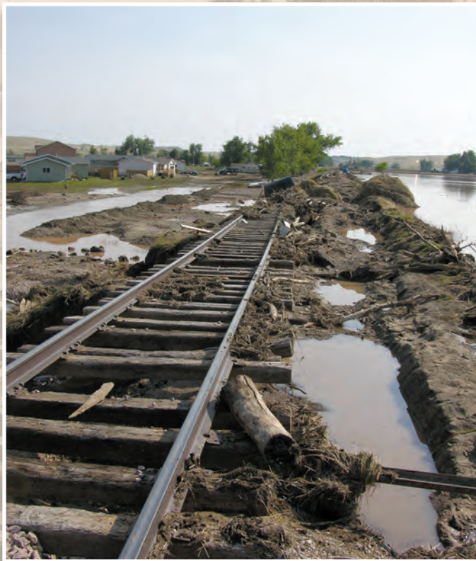
Figure 6. Photographs showing damages to houses and the railroad grade in the Hermosa area from flooding on August 17, 2007 (photographs by Mark T. Anderson).
