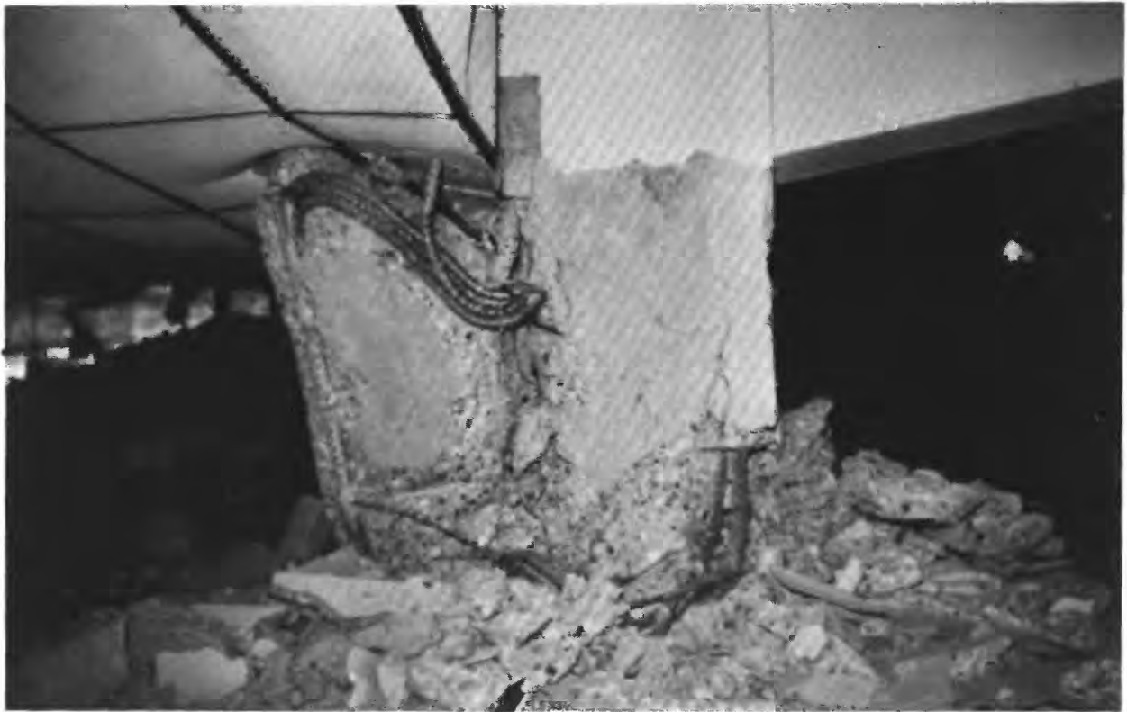
FIGURE 74.—Typical collapsed column in Hotel Terminal.
