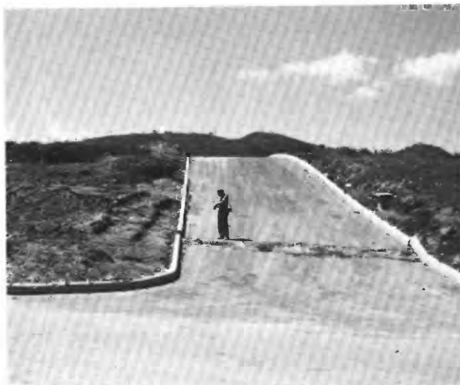
FIGURE 30.—Fault displacement of road at locality 1 (fig. 29). Note right-lateral component of displacement.
