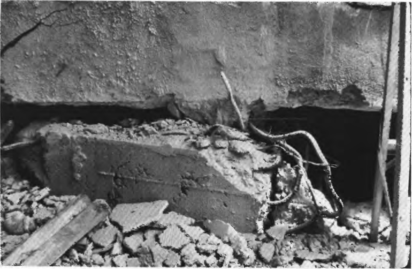
FIGURE 76.—Detail of column failure in second story at the Catholic Boys School. Story height now measured in inches.
