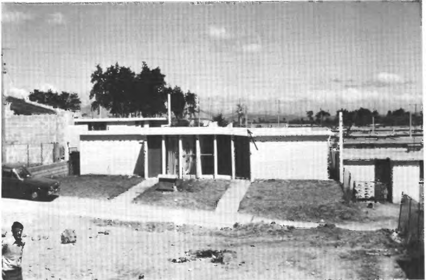
FIGURE 31.—Fault damage to a house in Guatemala City. The roof, foundation, and sidewalk have been displaced vertically.
