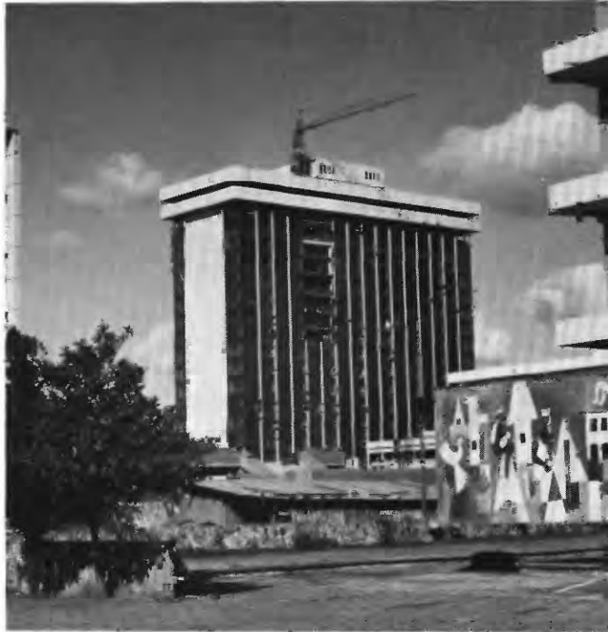
FIGURE 71.—The Finance Ministry Building (in Guatemala City) has 19 stories above ground plus 3 below. The undamaged steel-frame building is in the final stages of construction. (Photograph by W. H. Smith, American Iron and Steel Institute.)
