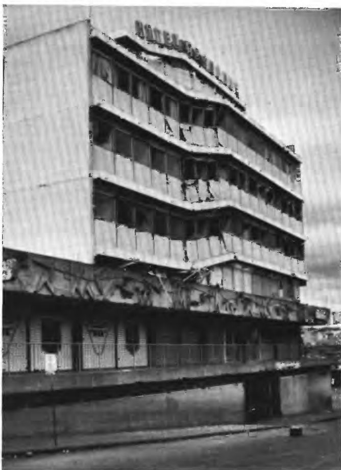
FIGURE 73.—Hotel Terminal in Guatemala City. Columns in third story collapsed.
