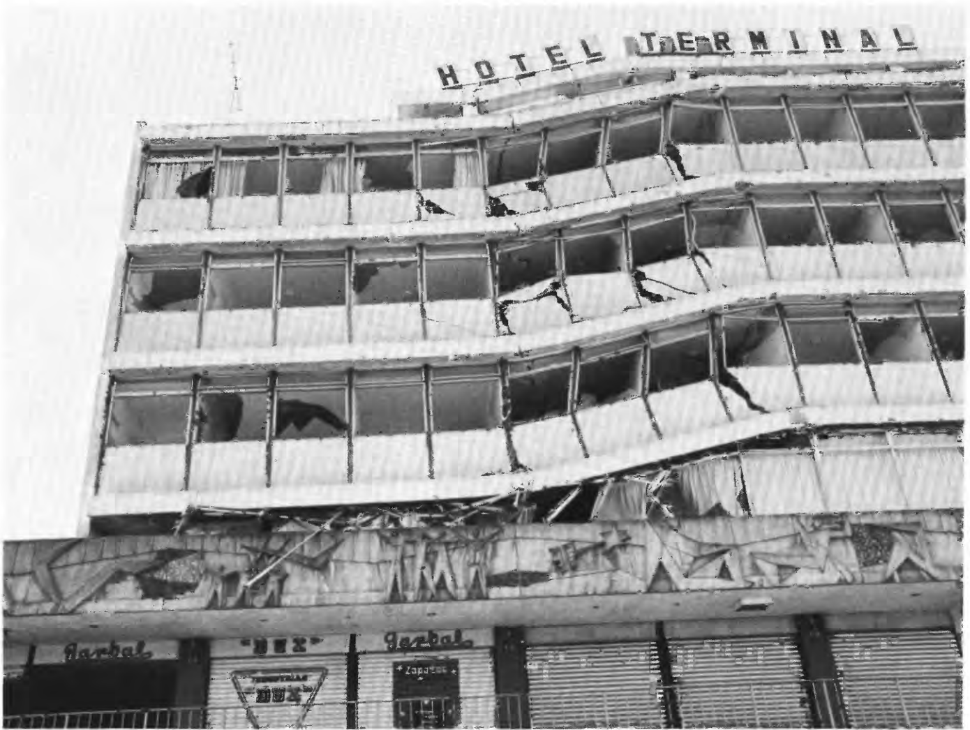
FIGURE 55.—Collapse of the Hotel Terminal, caused by the failure of reinforced-concrete columns in its third story. This building is located in Guatemala City (Zone 4).
