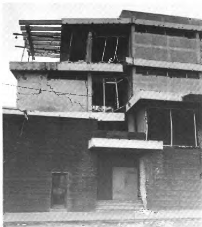
FIGURE 53.—Partial collapse of a three-story reinforced-concrete structure due to failure of columns in its second floor (Zone 12), Guatemala City.
