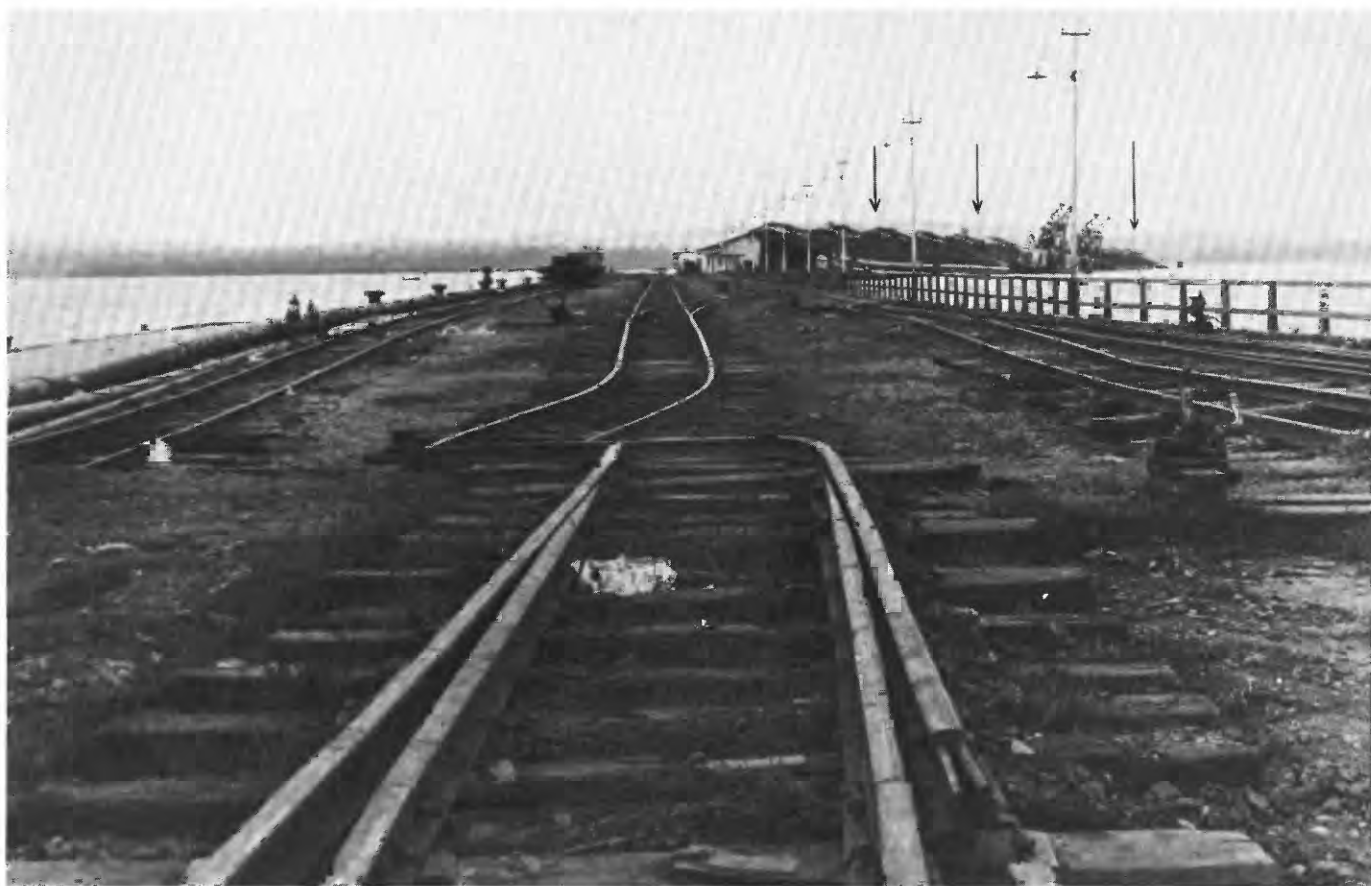
FIGURE 47.—Puerto Barrios wharf, Department of Izabal, destroyed by February 4 earthquake. Arrows show large warehouse partially submerged. See figure 40 for location of town.
