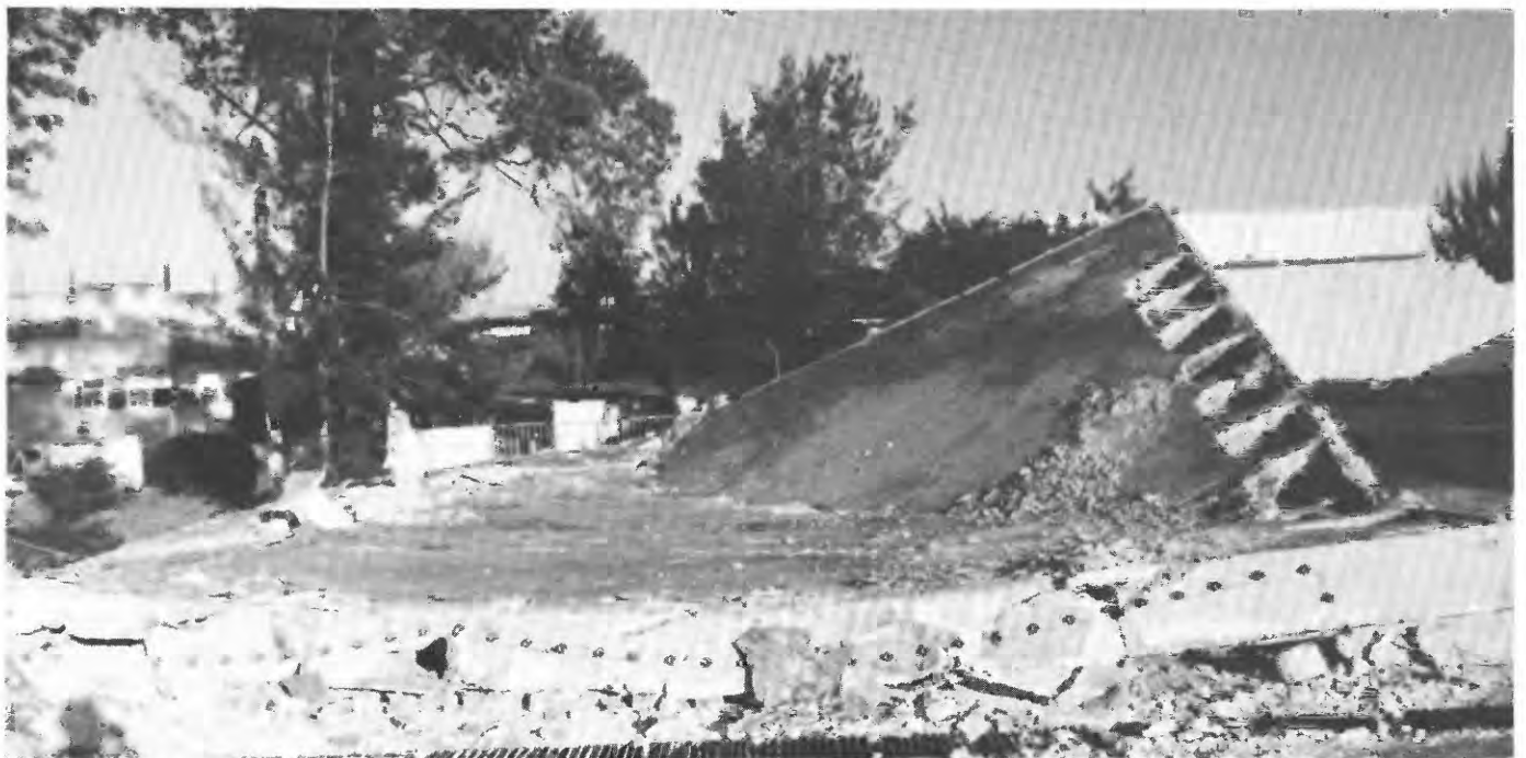
FIGURE 68.—Collapse of one-story reinforced-concrete framed structure in the Licorera Mixco, Mixco.
