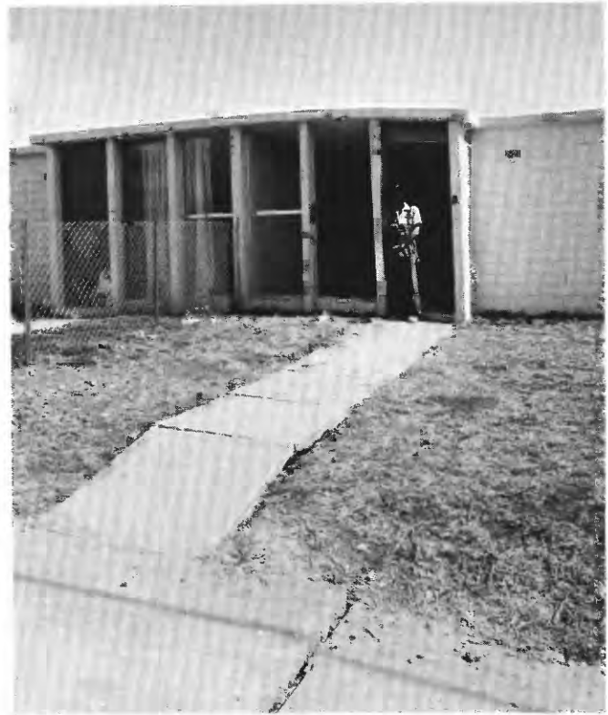
FIGURE 62.—Severe damage to reinforced-masonry construction caused by secondary faulting in Colonia San Francisco (Zone 19). The fault strikes north to northeast.
