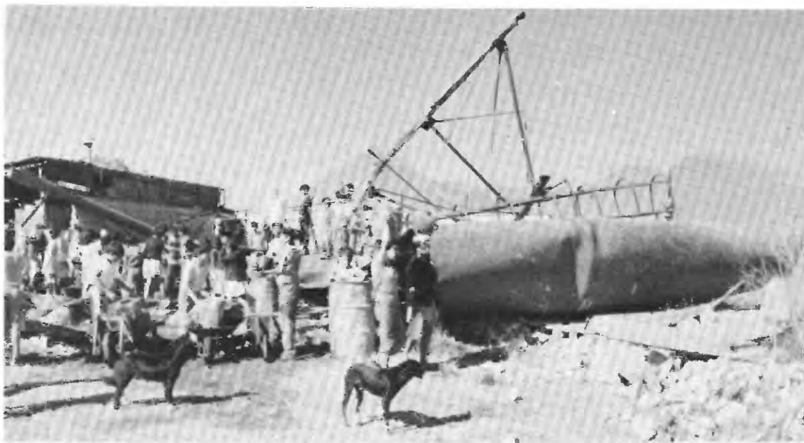
FIGURE 59.—Collapse of an elevated steel water tank in Villanueva, Colonia de los Planes, 22 km south of Guatemala City.
