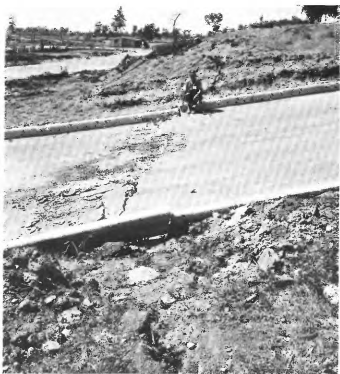
FIGURE 63.—Rupture across the San José Rosario subdivision. Fault with 13 cm vertical and 5 cm right-lateral displacements (Zone 19).
