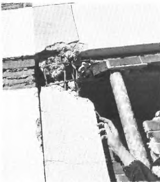
FIGURE 66.—Failure of short column in three-story framed reinforced-concrete structure in Guatemala City (Zone 7).
