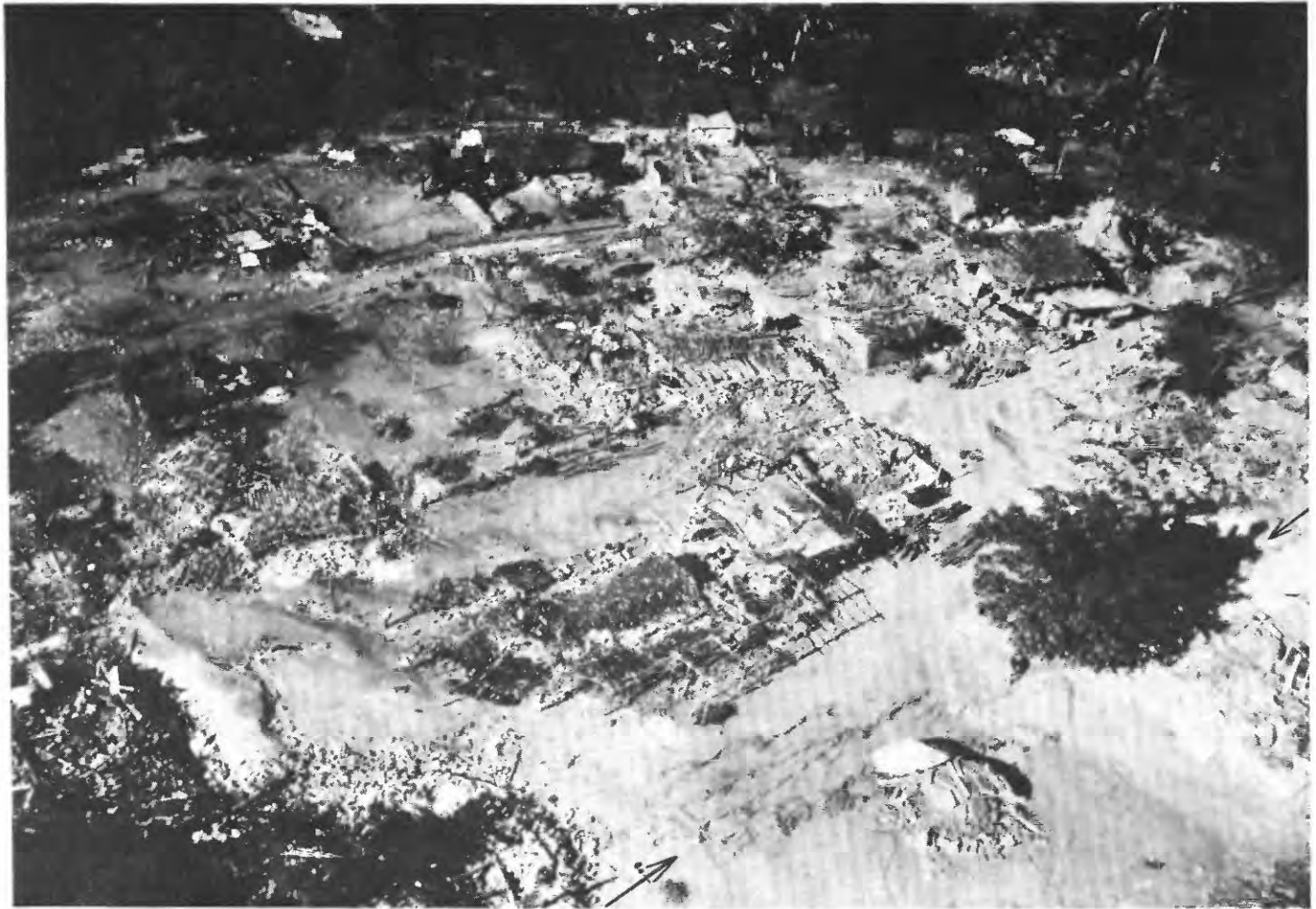
FIGURE 28.—Part of the village of Subinal, 7 km west of El Progreso, showing the destruction of adobe structures near the Motagua fault trace. The fault is a broad zone of ground cracks that cuts diagonally across the lower right corner of the photograph (arrows).
