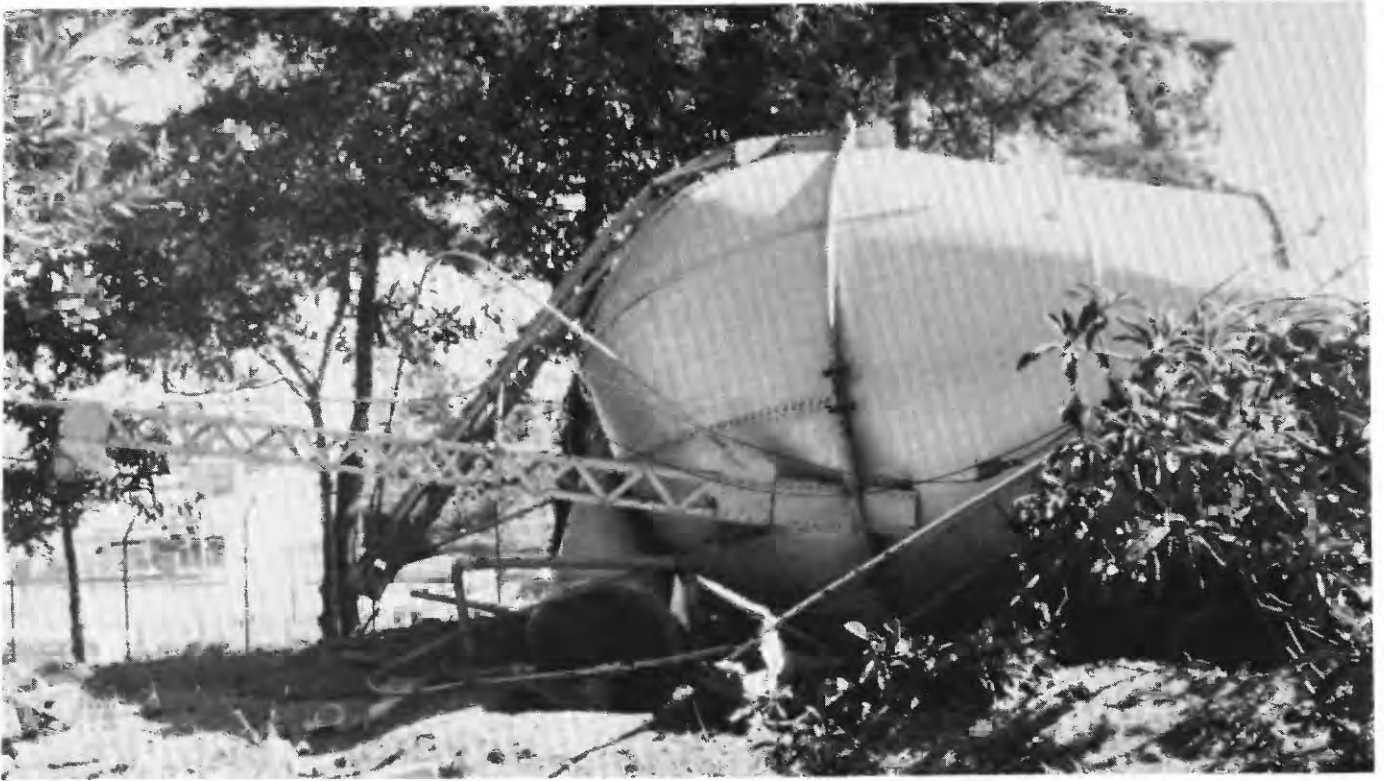
FIGURE 57.—Collapse of an elevated steel water tank in the Instituto Técnico Vocacional in Guatemala City (Zone 13).
