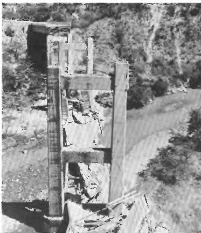
FIGURE 64.—Collapse of three central spans of the Agua Caliente Bridge, Kilometre 36 on the road to the Atlantic Ocean. This bridge was constructed in 1959.
