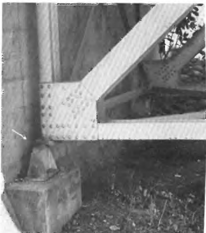
FIGURE 65.—Benque Viejo Bridge, on the verge of collapse after failure of supports, shown by arrow.
