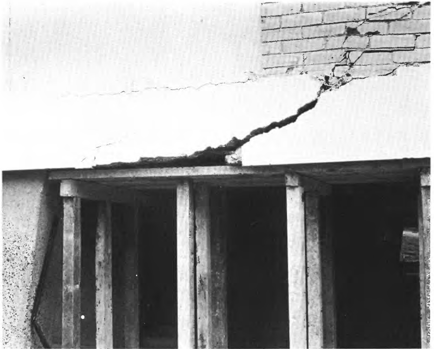
FIGURE 70.—Severe damage to flat beams and slab in the five-story reinforced-concrete Edificio ELGIN, in Guatemala City (Zone 14).
