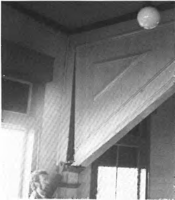
FIGURE 51.—Damage to a wooden structure in Puerto Barrios, caused in part by ground compaction. Note the large offset of 11 cm shown in the photograph.
