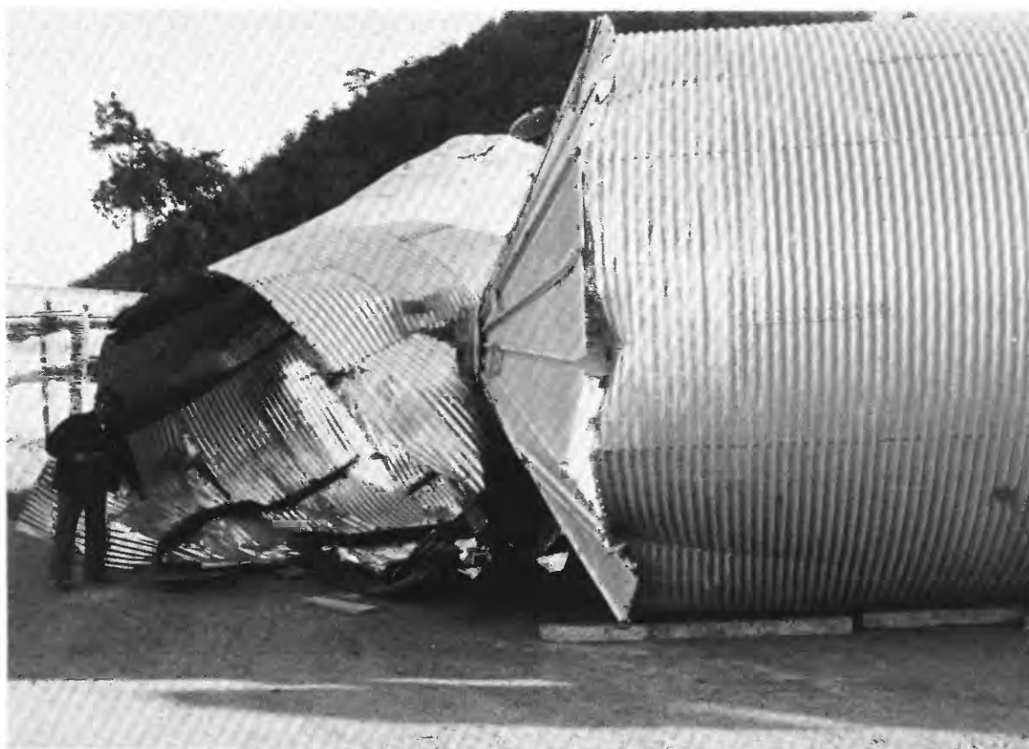
FIGURE 60.—Collapse of a corrugated-steel grain silo in Villalobos, 5 km southeast of Guatemala City.
