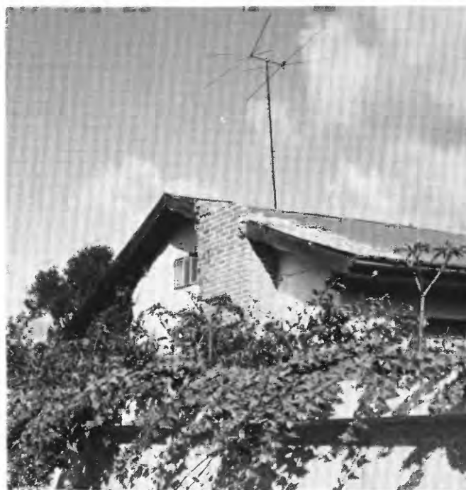
FIGURE 48.—Chimney collapse from a one-story house in Guatemala City, Zone 11.
