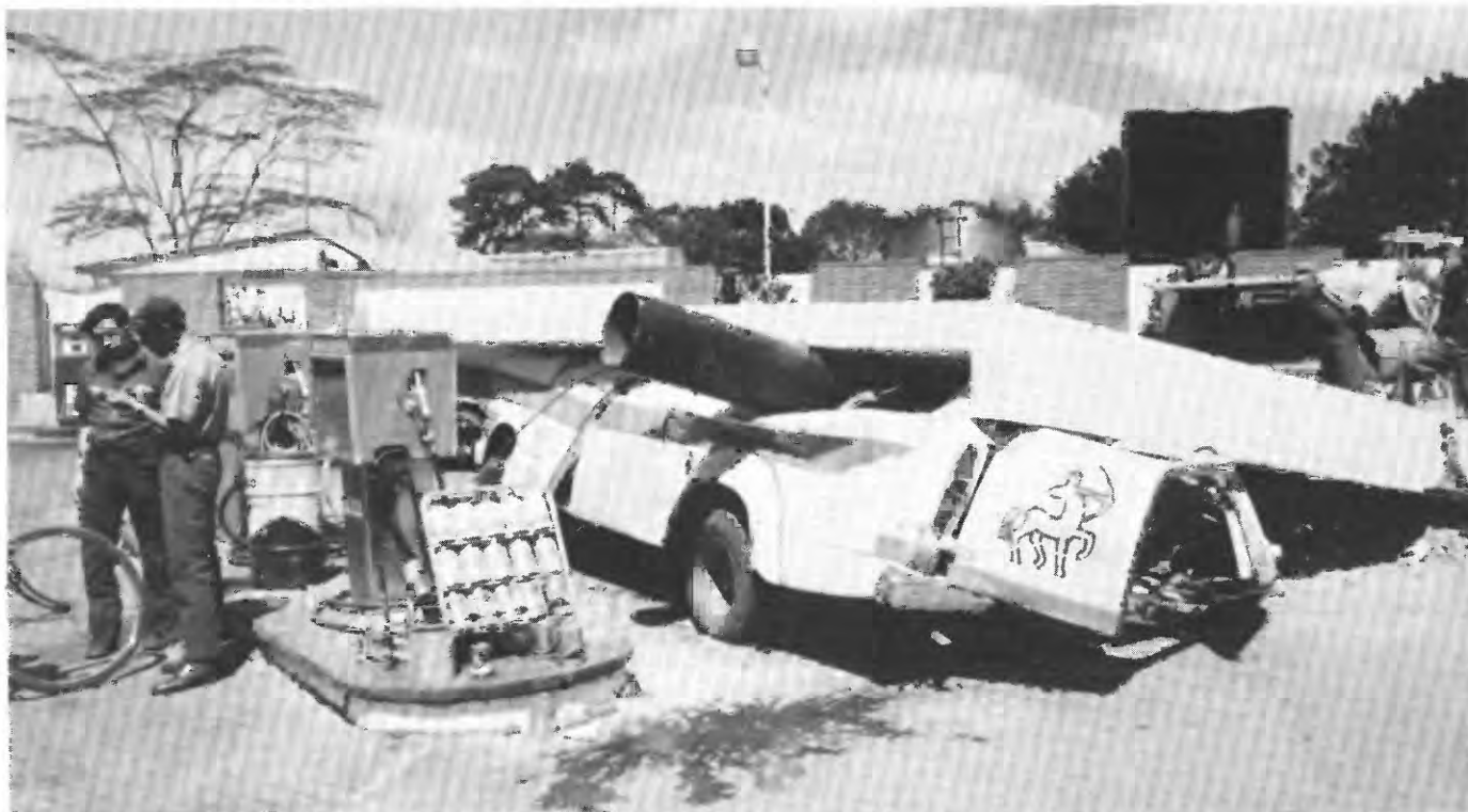
FIGURE 56.—Collapse of inverted-pendulum gas-station structure, Guatemala City (Zone 7).
