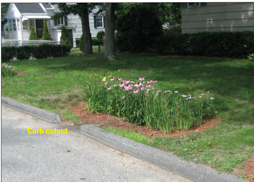
Figure 9. Low-impact-development (LID) features installed in the LID-retrofit neighborhood along Dexter Street and Silver Lake Avenue, Wilmington, MA.
