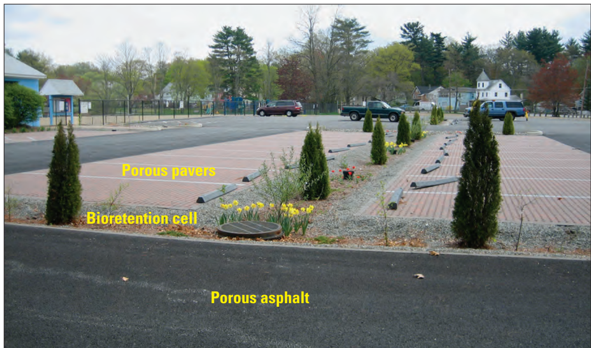
Figure 2. Low-impact-development features installed in the parking lot at Silver Lake Beach, Wilmington, MA.
