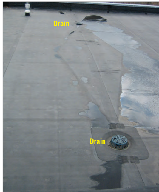
Figure 16. The conventional, rubberized-membrane roof on the Ipswich, MA, Town Hall.
