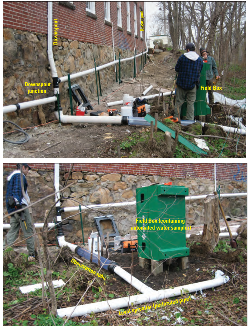
Figure 17. The system, during construction, for collecting stormwater runoff from the Whipple Annex green roof, Ipswich, MA.
