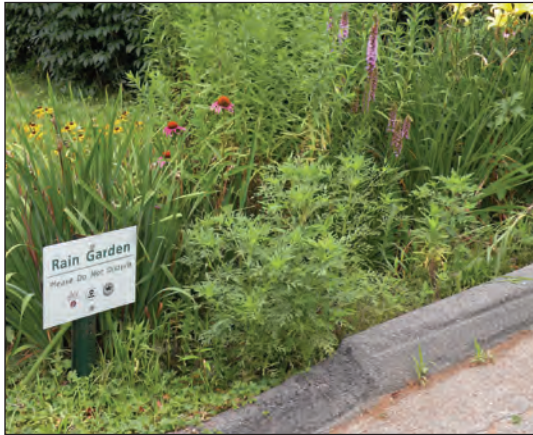
Rain garden designed to enhance infiltration at Dexter Street, Wilmington, MA.
