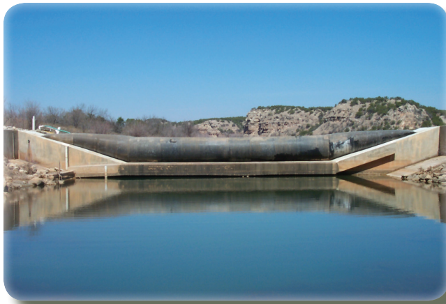
Figure 2. Upstream view of inflated low-flow collection dam, South Wichita River near Guthrie, Texas.
