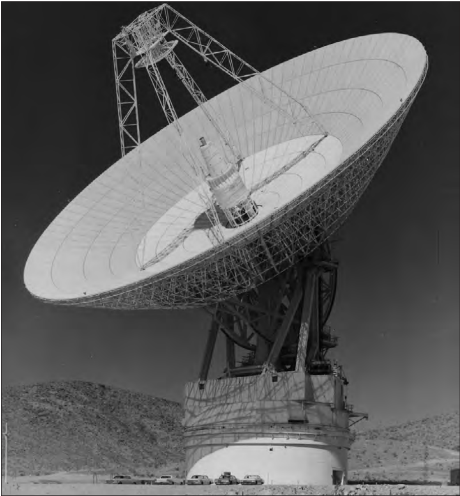
NASA/JPL's new 210-ft diameter antenna at Goldstone, California: April 1966 (Photo: NASA/JPL-Caltech Archives, Photo number 332-9278Bc).
