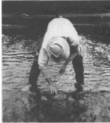
Research technician preparing silt traps by washing gravel in running water to remove "lines" (ca. 1957) (luneau 557)
