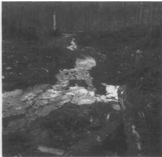
Watershed study on the Harris River, spur 241. The drainage was first cat-logged, then the creek was diverted, the gravel removed and finally, the creek re-diverted to its original course minus the gravel. Photo taken in 1959 (Juneau 567)
