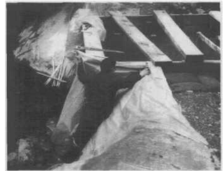
Doug Swanston wrestles a sheet of plastic into place during the construction of the collection basin for the flume at Young Bay Experimental Forest. The flume provided watershed research with a stream bed that could be manipulated to simulate a variety of conditions. (Helmerts collection)
