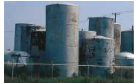
Figure 4. Abandoned tanks and pipes may contain radium in scale and sludge.
